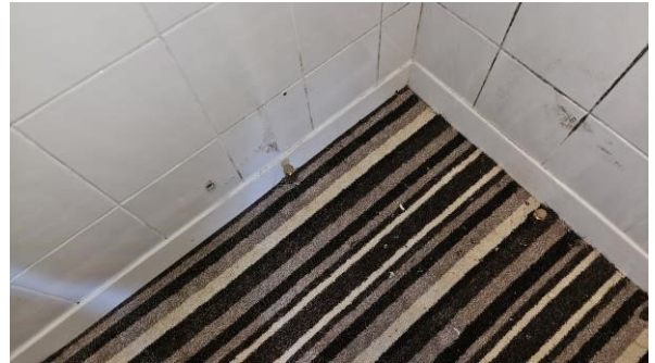
12 Pipework tails above floor level.
