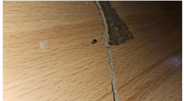
20 Example of panel pin protrusion above veneer height creating safety hazard.
