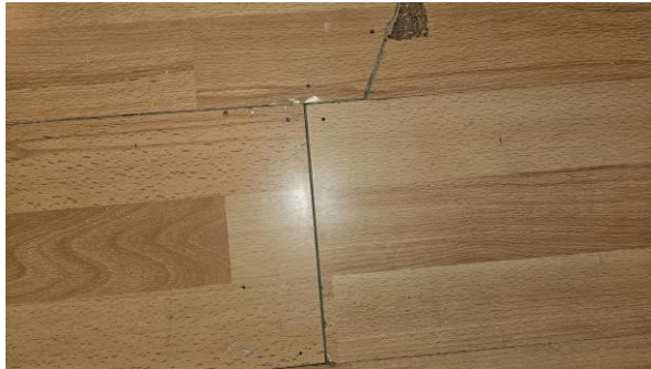
19 Hall – split plank and various panel pin fixings.
