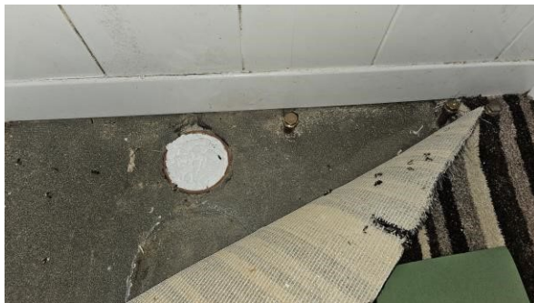
13 Poor silicon sealant capping to soil pipe.
