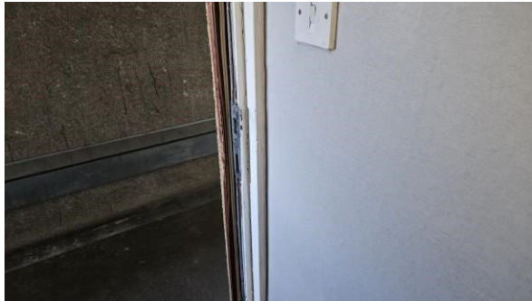
9 Front door – defective door stop.
