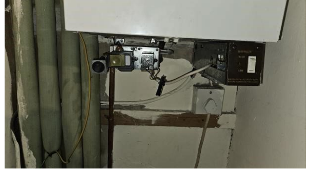
2 Gas fired boiler not operational.
