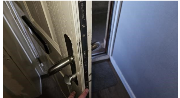
8 Front door defective locking mechanism.
