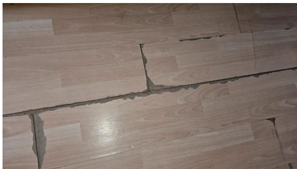
21 Main Bedroom – failed floor covering.
