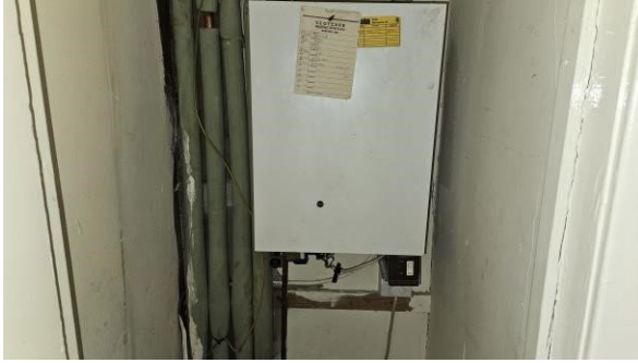
1 Gas fired boiler not operational.
