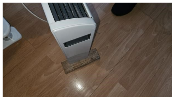
24 Portable convector heater – inappropriate
