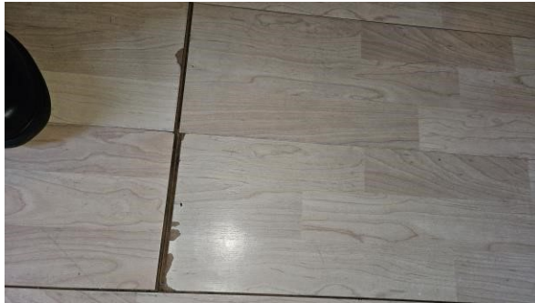
17 Second Bedroom – sliding of planks and unsecured pin fixing joints.
