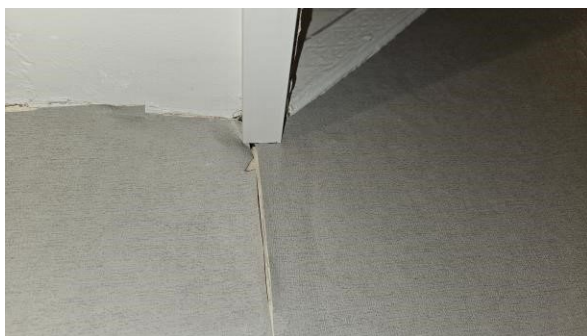
15 Minor damage at circulation corridor adjacent to with cabling penetration.
