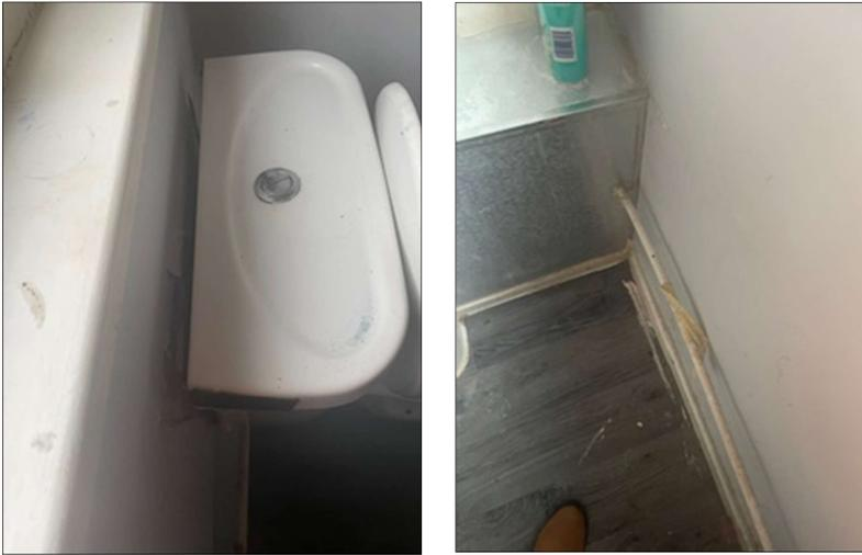
The toilet cistern has come away from the wall and the overflow pipe has been sealed with masking tape no leaks were noted - No repairs carried out.
