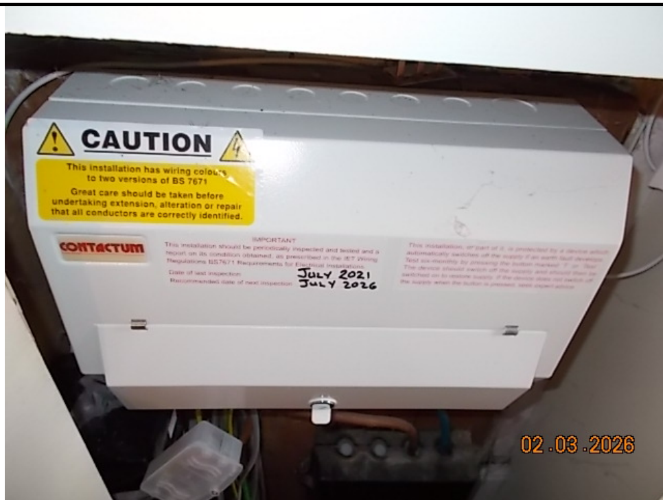
19. Testing record on Consumer Control Unit
