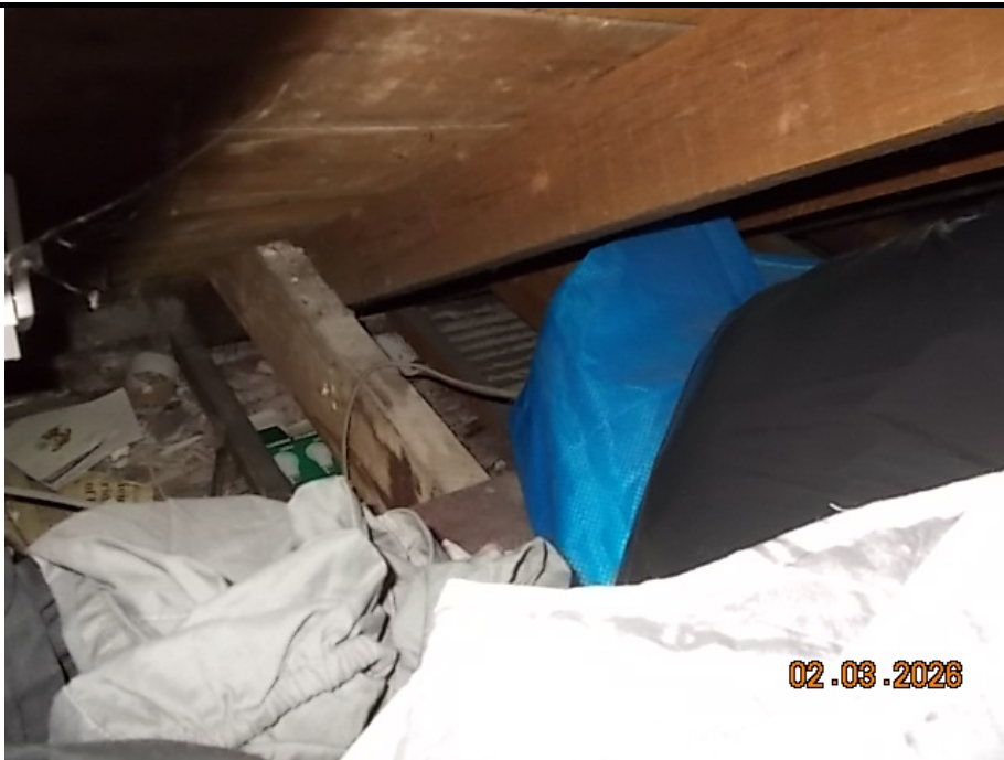
24. Eaves Roof void from Stair
