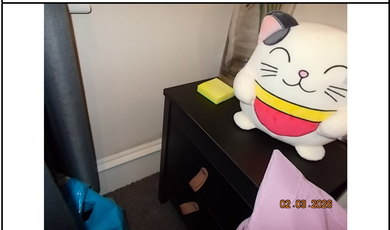
14. Front Bedroom corner of outer walls
