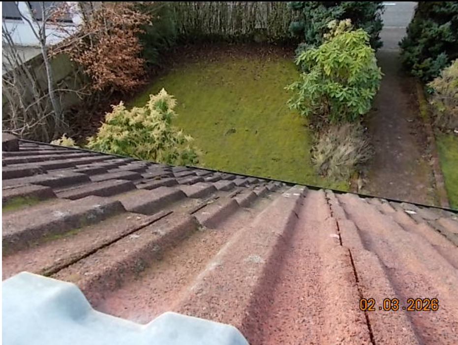
23. Front roof slope from First Floor Front Bedroom
