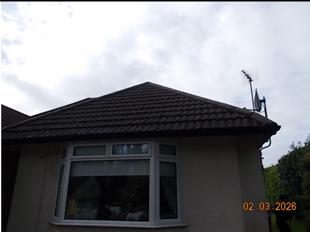
30. Rear Bedroom Roof
