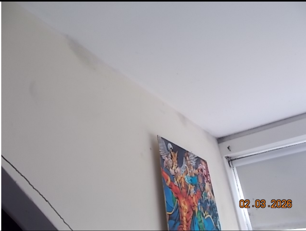
21. First Floor Front Bedroom Dormer Cheek
