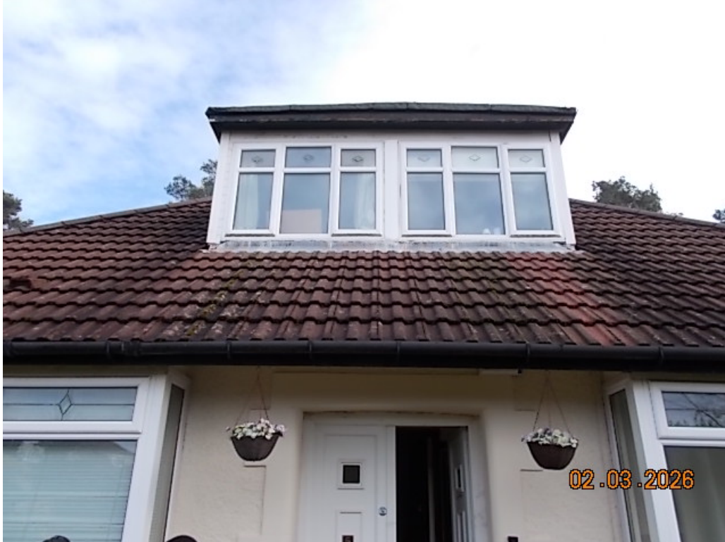
27. First Floor Front Bedroom Dormer window
