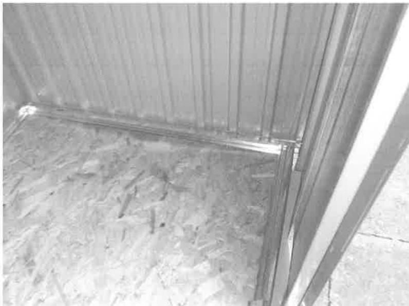
6. Replacement shed – gaps at floor junction and water puddling on floor
