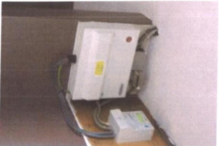
4) New electric consumer unit and upgraded fire detection system as at 24/03/017
