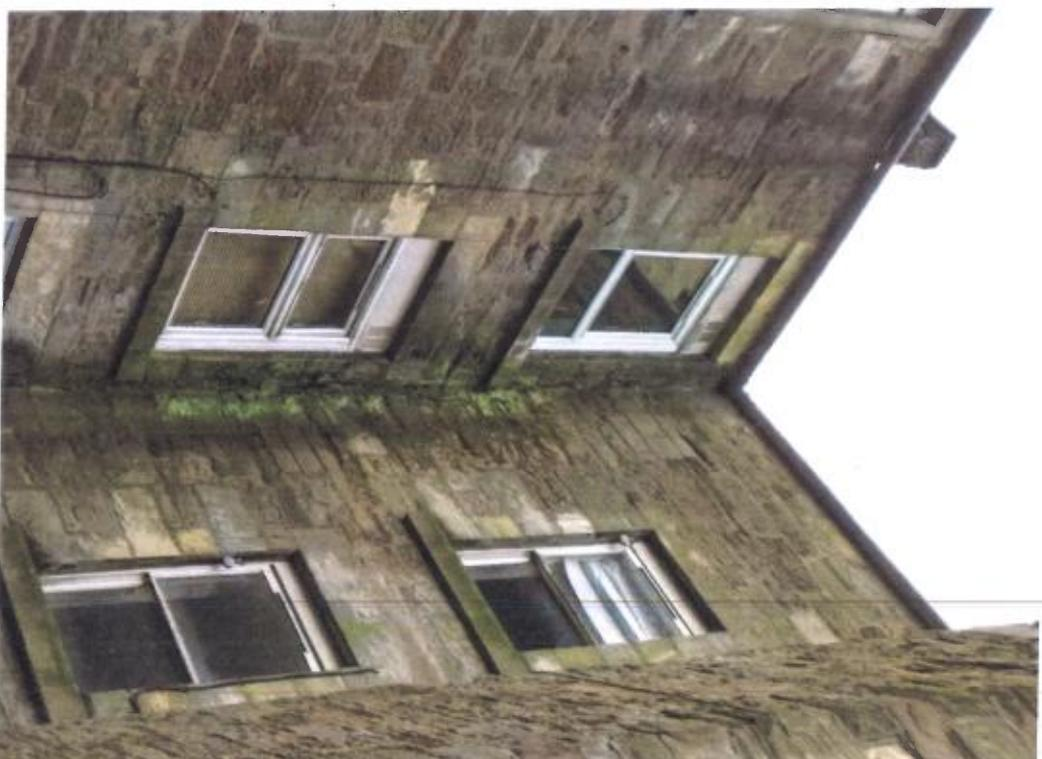
As/10/17: gutters have been cleared and appear to be in working order. Plant growth has been removed from the wall.
