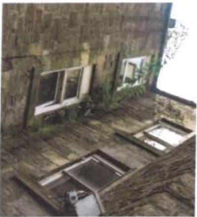
As at 3/07/17: gutters blocked with plants, extensive growth from crevices in wall
