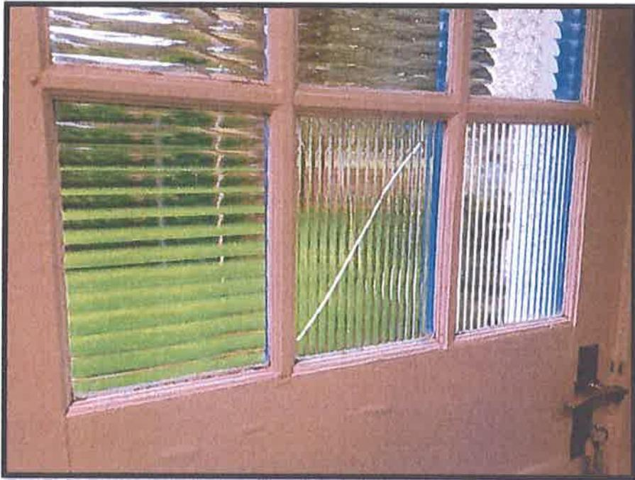
Photograph 14 Cracked pane to rear door window.
