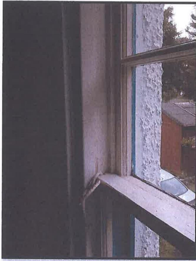
Photograph 12 Rear double bedroom window - broken sash cord.
