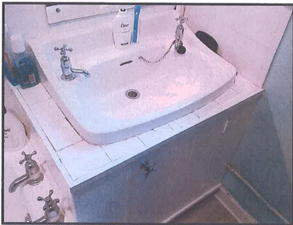
Photograph 8 Cracked tiles around wash-hand basin.
