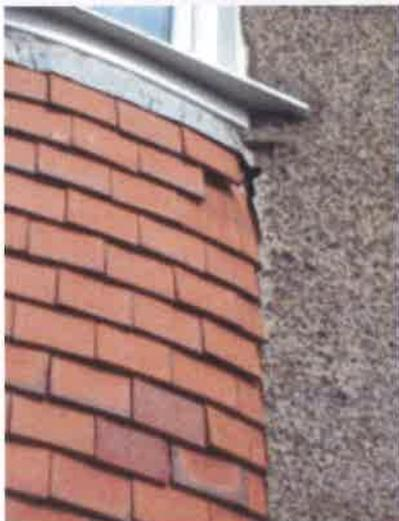
Front Elevation - slight damage to roughcast right side of oriel window
