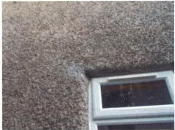
Rear Elevation - example of historic cracking at lintels
