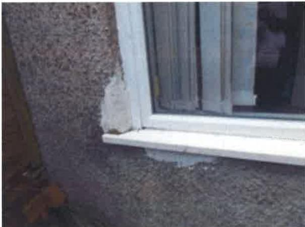
Rear Elevation - Roughcast patched - side of box room window
