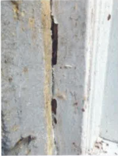
Rot to external timber door facing - left side of new front door
