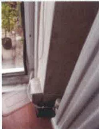
Internal - Living room window - slight staining from former leak/ minor redecoration required
