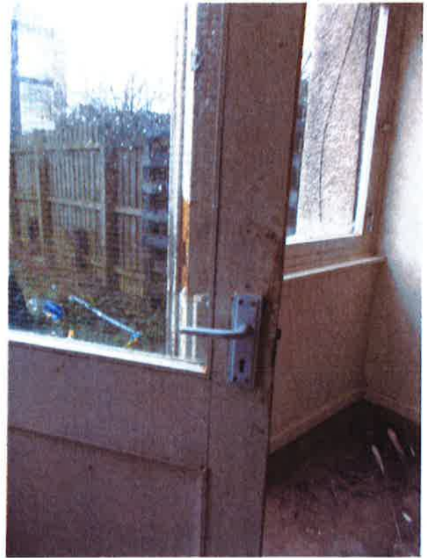
1.(j) New mortice lock to back door - internal
