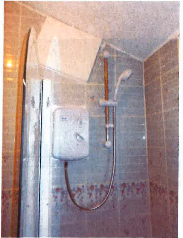
14. Bathroom - Repair to tiled wall above shower
