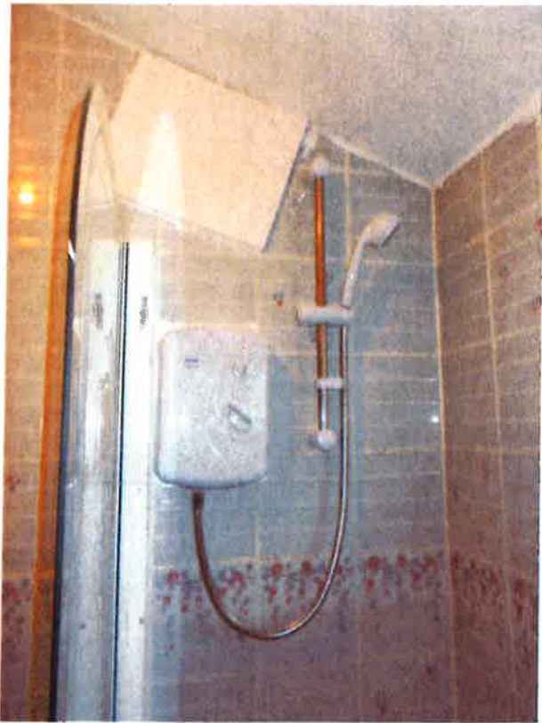
4. Shower complete and functioning
