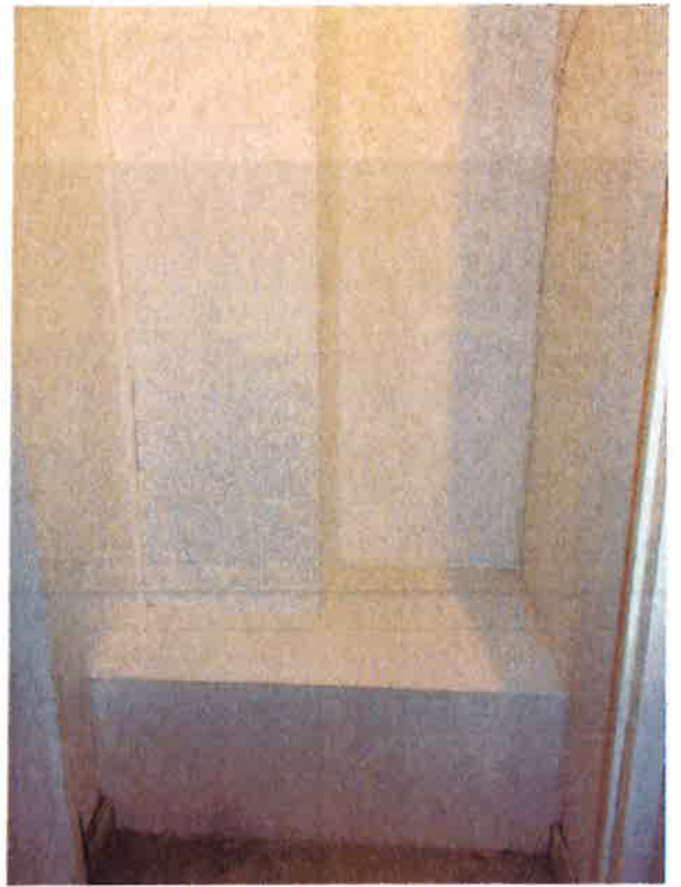
1. (e) Cupboard - 1st floor landing adjacent to room with boiler
