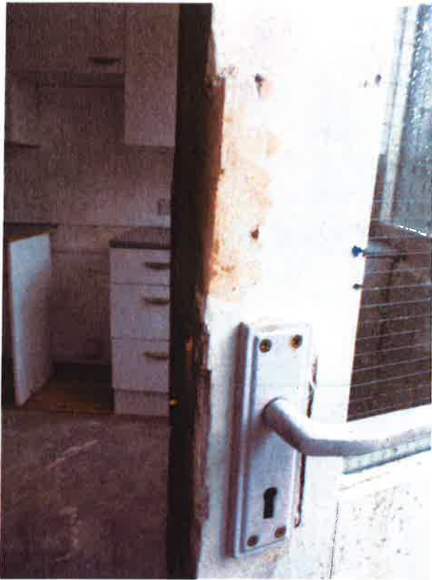
1. (j) New mortice lock to back door external
