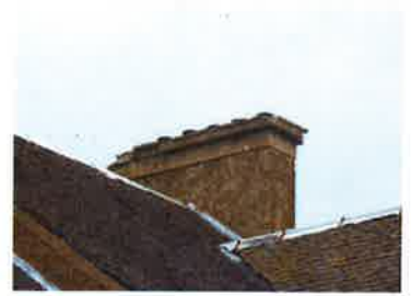
7. Roof and chimney - back
