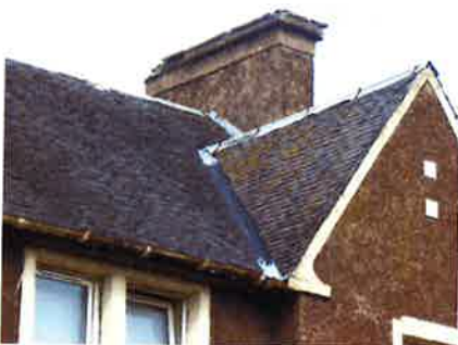
2. Roof and chimney - front
