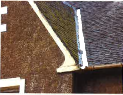
5. Repair to valley gutter
