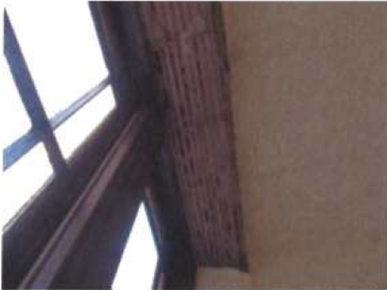
Landing Window/Ceiling between 1st and 2nd Floor
