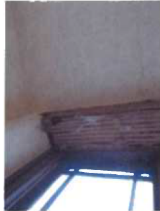
Landing Window/Ceiling between 1st and 2nd Floor
