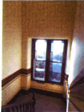
4) The ceiling above the window on the landing between the first and second floors of the tenement has not been repaired or replaced. The internal fabric of the close walls and ceiling are continuing to deteriorate.
