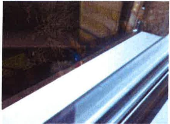
Communal close window to top landing - gap at side of external sill
