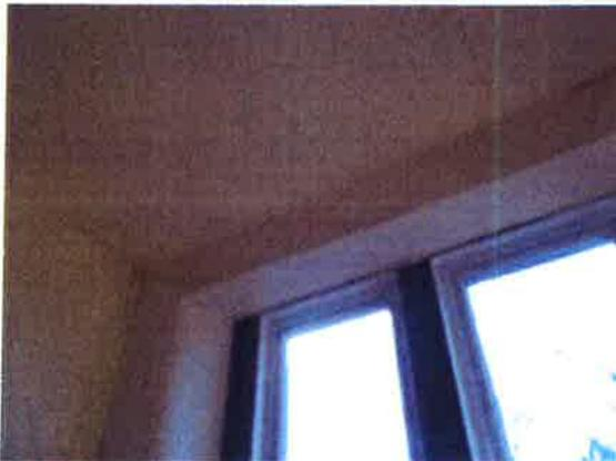
Communal close window to middle landing - plaster repaired above window. Cracks to ceiling and wall.
