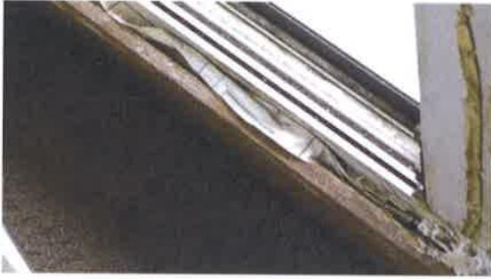
Photo 2 – Damaged facing at balcony door
