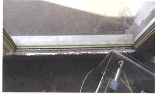
Photo 3 – Defective sealant on frame
