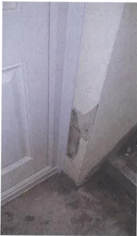
Photo 8 – New door installation damage
