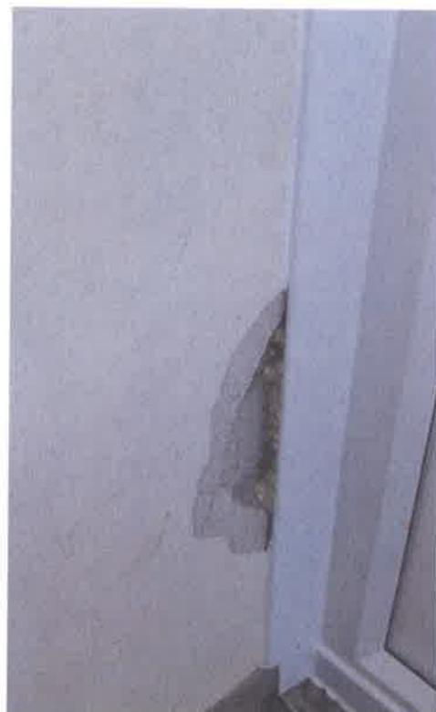
Photo 9 – New door installation damage
