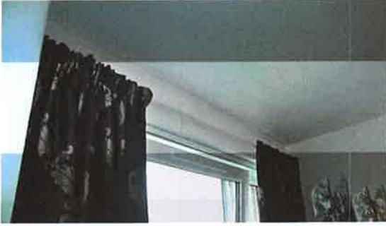
**Photo 8** – Bed 1. Damp and mould on ceiling
