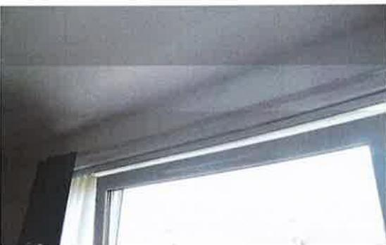
**Photo 6** – Bed 2. Damp and mould on ceiling
