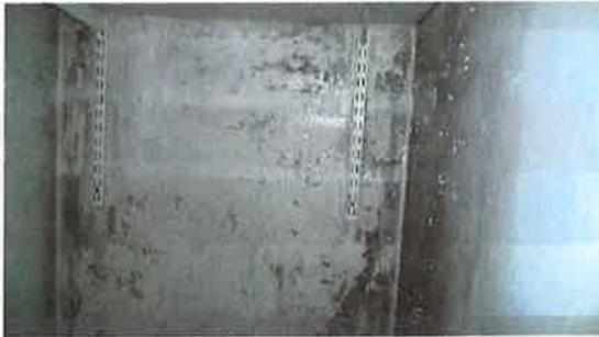
**Photo 10** – Bed 1. Saturated wall in press
