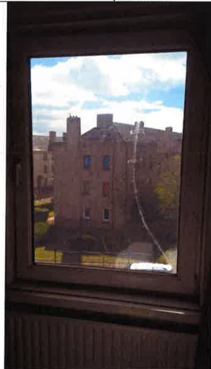
Front bedroom window. Double glazed unit cracked with inoperable closing mechanism. Requires to be replaced.
