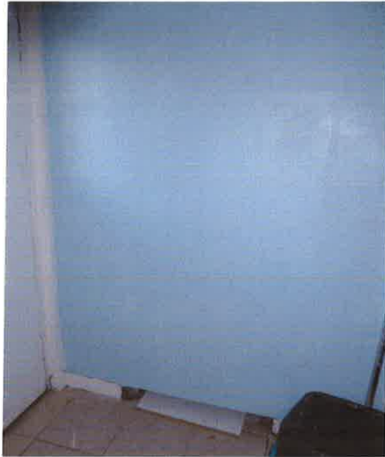
Ex-alcove cupboard to kitchen – reinstate
