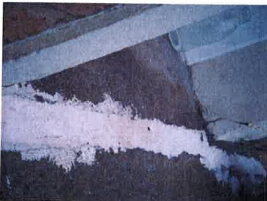
Repair carried out to step, however the durability of the repair cannot be comment on as the product used to repair is unknown.
