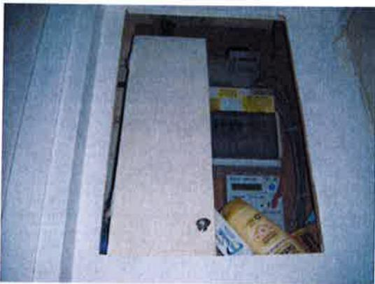
Door to cupboard missing, tenant unable to produce door to be rehung by contractor.
