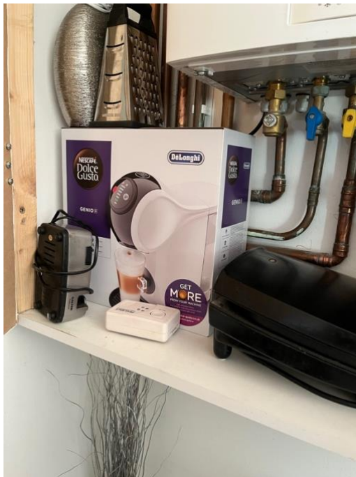
Photograph 7: Carbon monoxide detector on shelf beneath boiler
