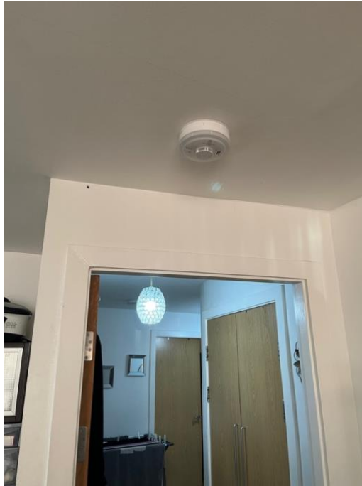
Photograph 8: Heat detector – living room
