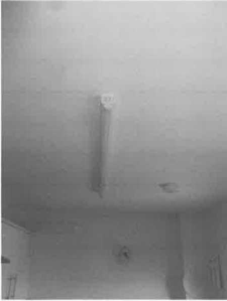
New light fitting in kitchen and heat detector – April 2018
