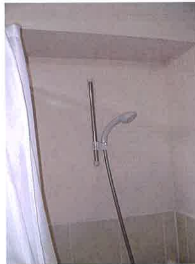
Photo 9 – Showerhead in main bathroom
