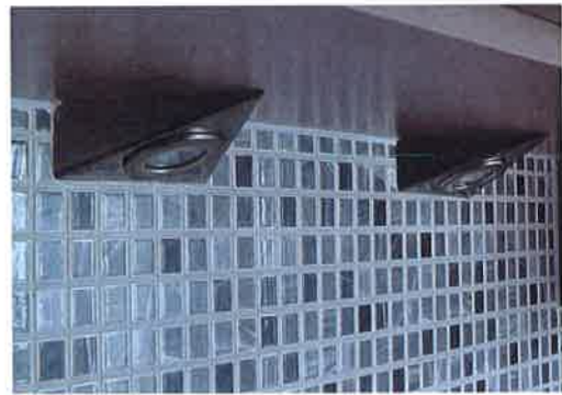
Photo 7 – Kitchen worktop lights
