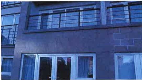
Photo 4 – Balcony above living room
