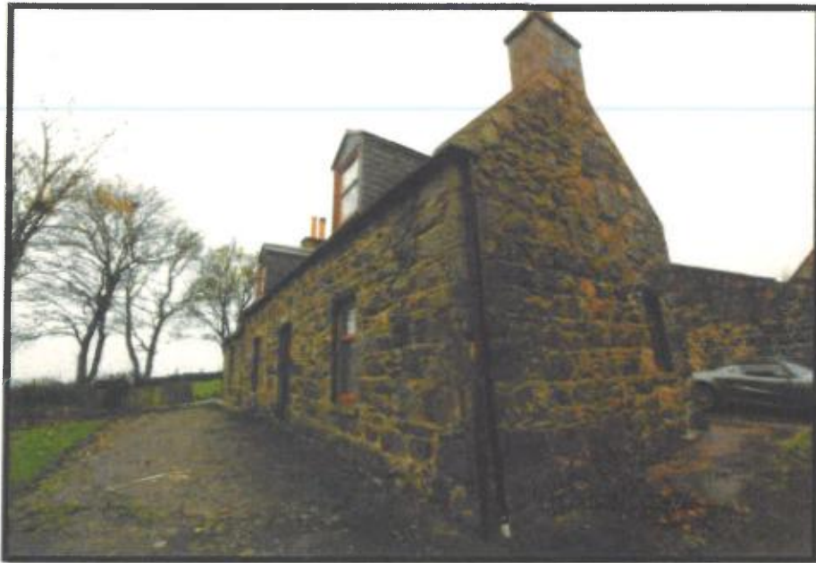
Figure 3 Front corner - Gutters replaced.
