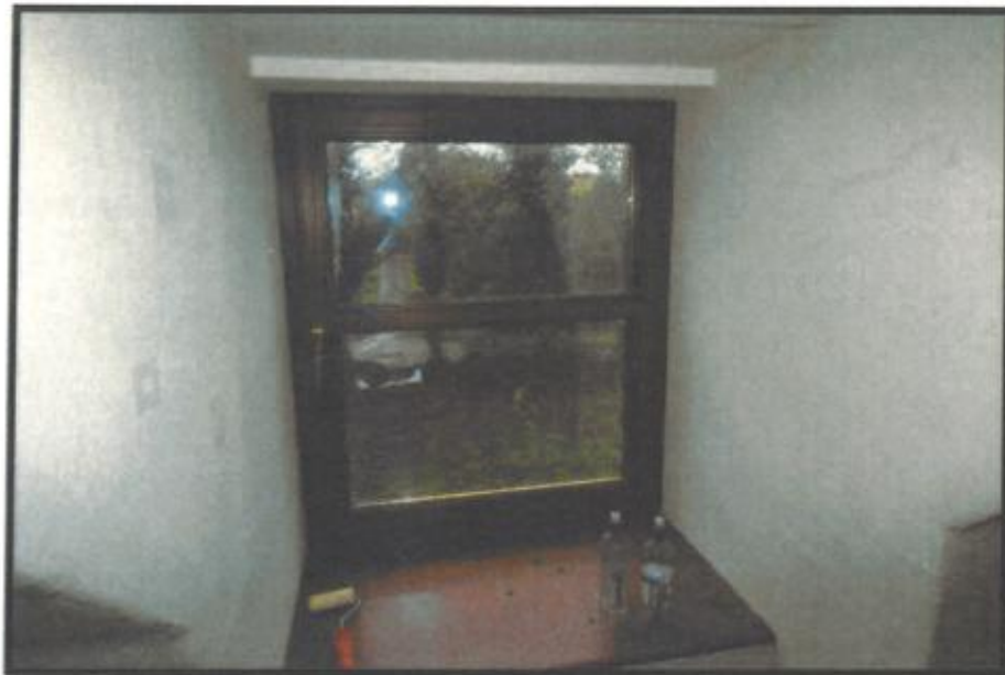
Figure 11 Right first floor bedroom window internal.
