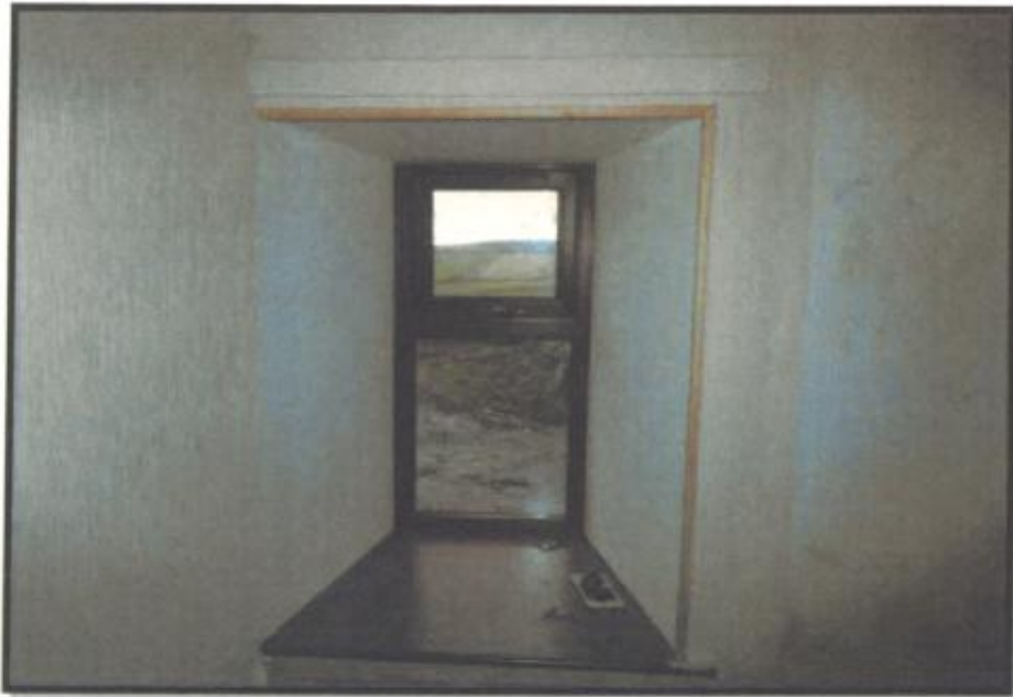
Figure 10- Right ground floor bedroom gable window internal - typical finish.
