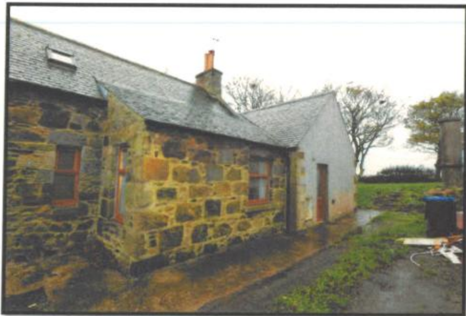
Figure 7 Rear elevation - windows and guttering replaced.
