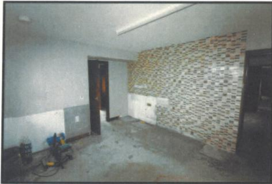
Figure 9 ~ Kitchen units stripped out, stove removed.
