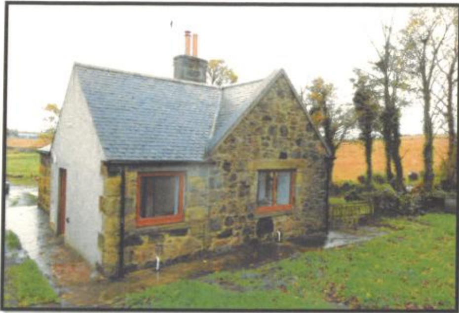
Figure 6 Left gable elevation/side addition - Windows and gutters replaced.
