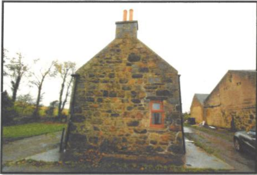
Figure 2 Right hand gable elevation - cracks re-pointed, window replaced.
