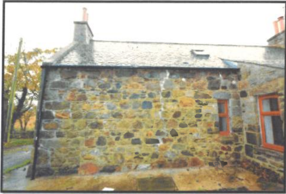
Figure 8 Rear left corner - both cracked areas re-pointed, windows and guttering replaced.
