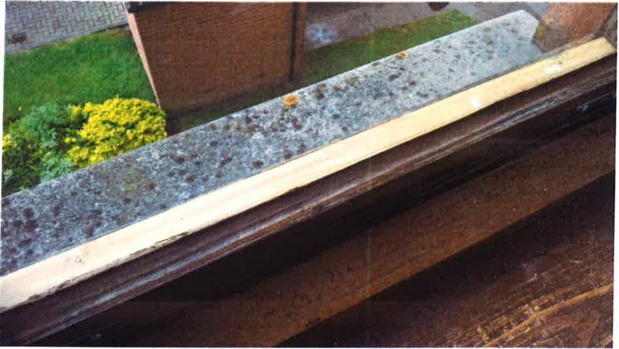
5. View of remedial works completed, new timber bead, angle brackets etc.
