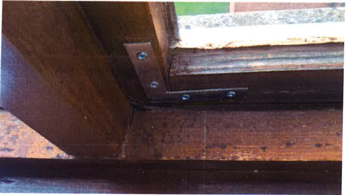
7. Close view of angle bracket and sealant remedial works.
