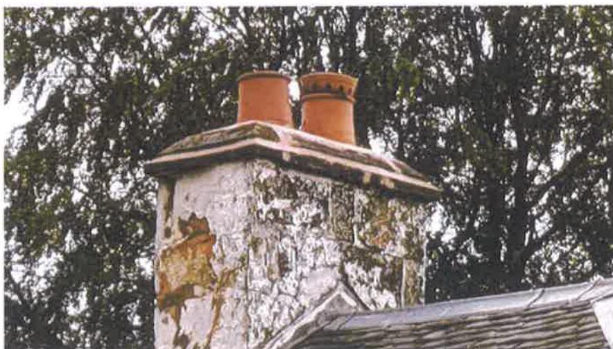
2 The repaired chimney
