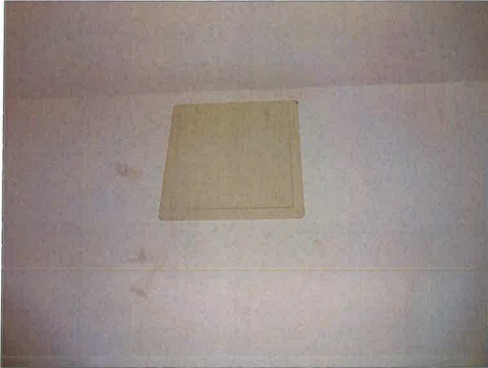
Hallway – hole in wall now repaired and access hatch fitted
