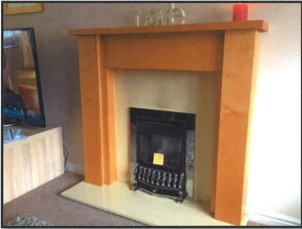
Figure 2 Gas fire in Lounge
