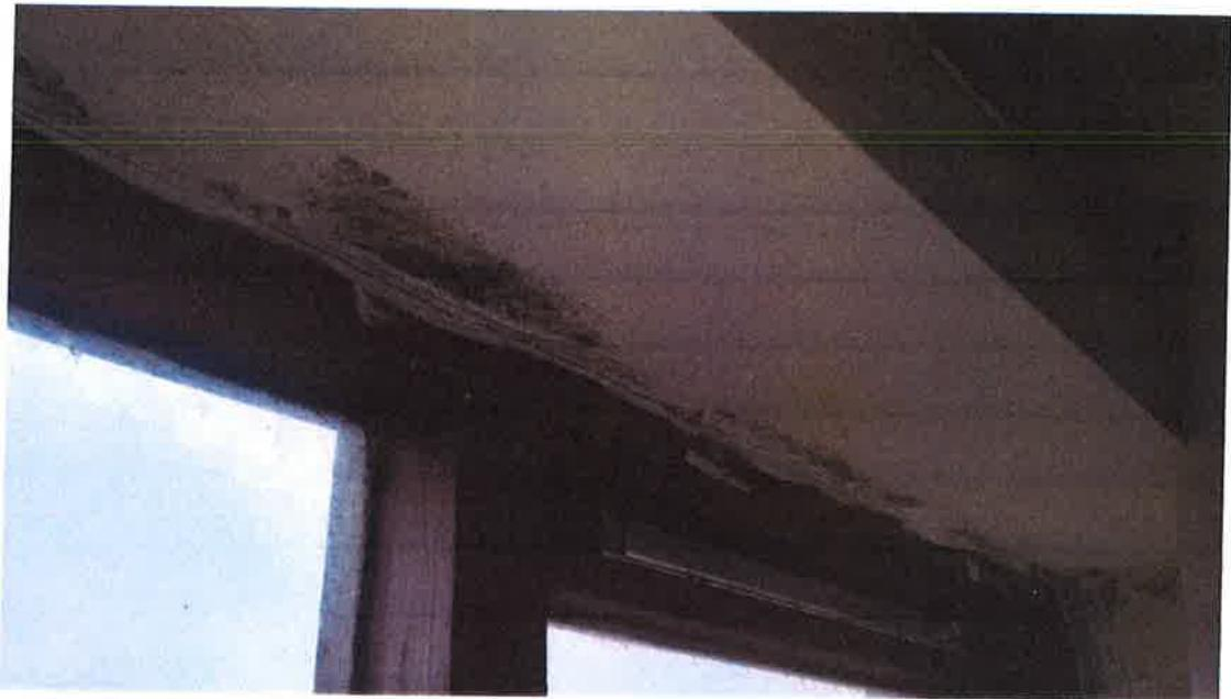
2. Living Room window soffit – mould growth to lining.
