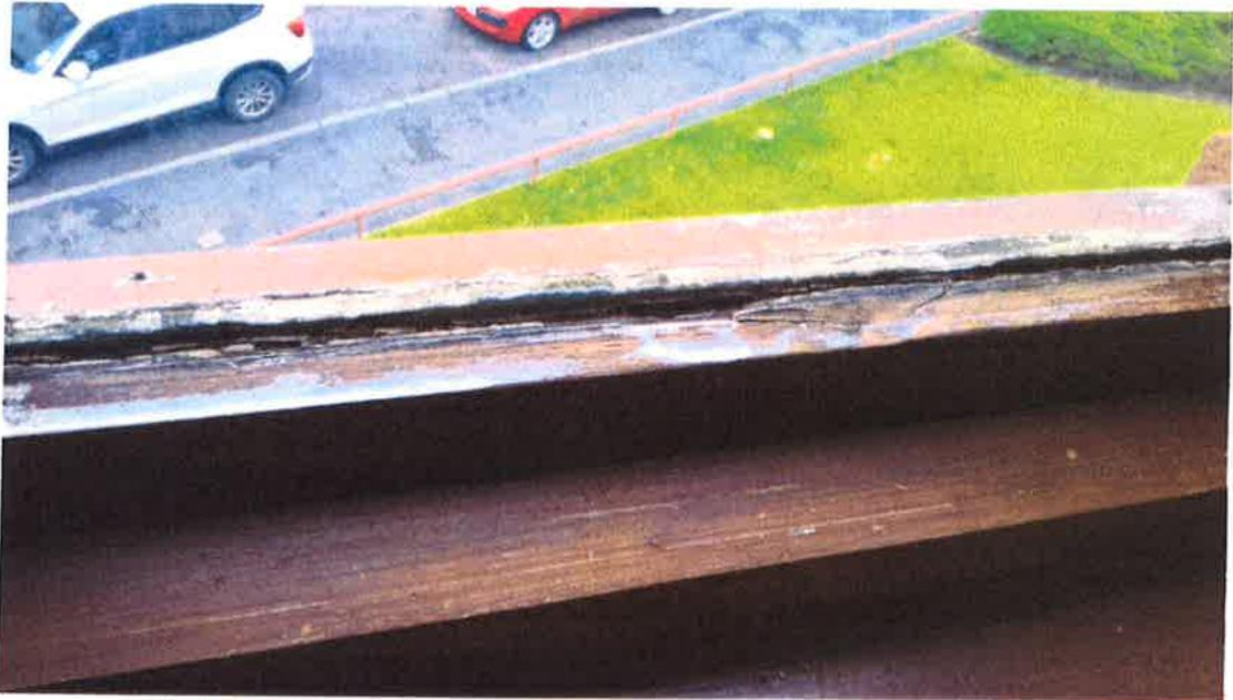
5. Close view of defective glazing putties, water ingress at seal and timber decay to window frame.
