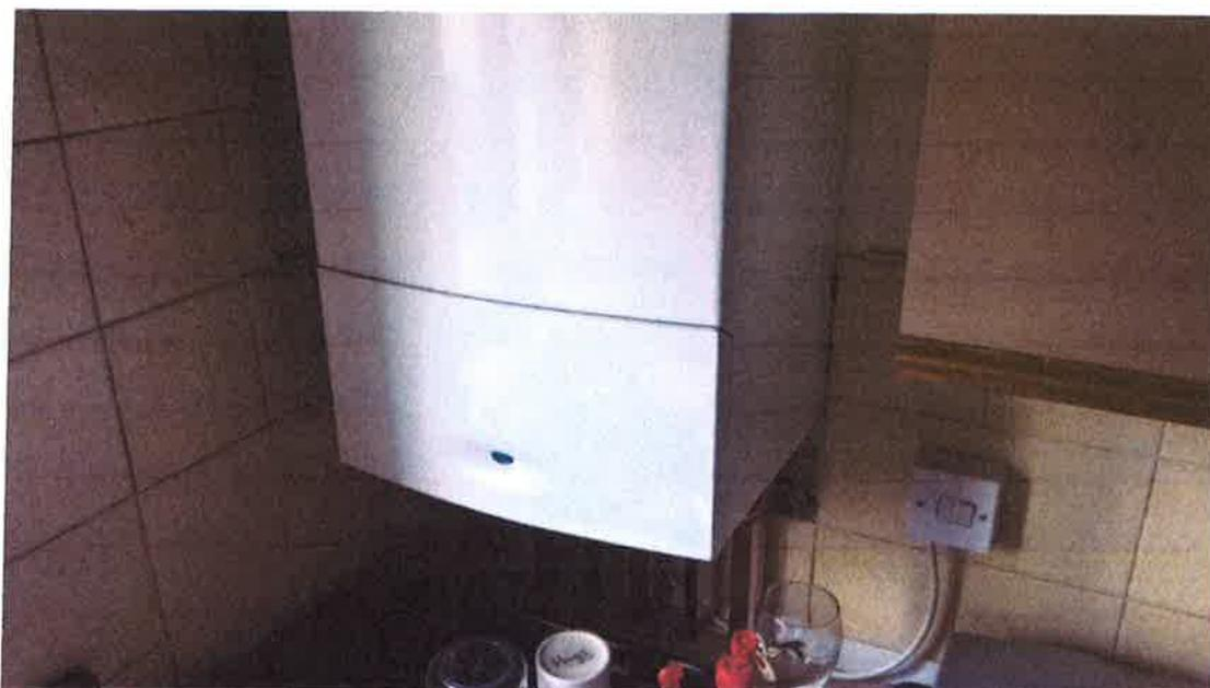
9. Gas boiler within Kitchen – no evidence of maintenance, servicing or a Gas Safety Certificate.
