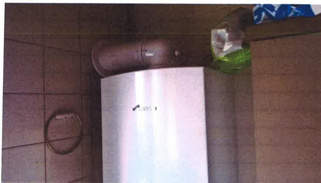
10. Gas Boiler – no evidence of any carbon monoxide detector within Kitchen.
