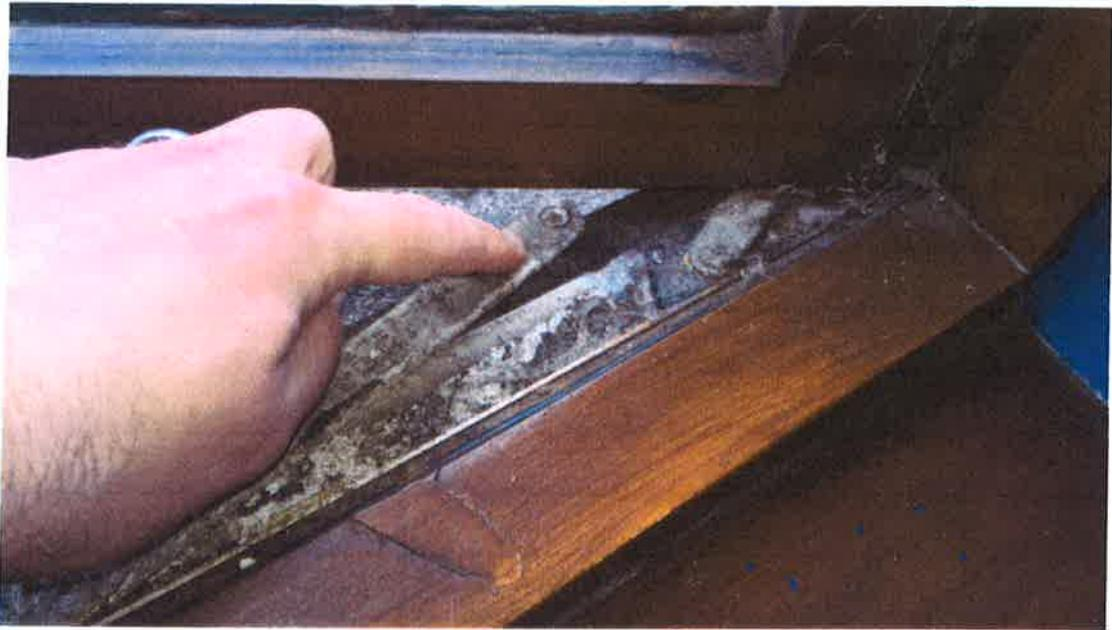
**7. Window casement hinge not secured to window**
