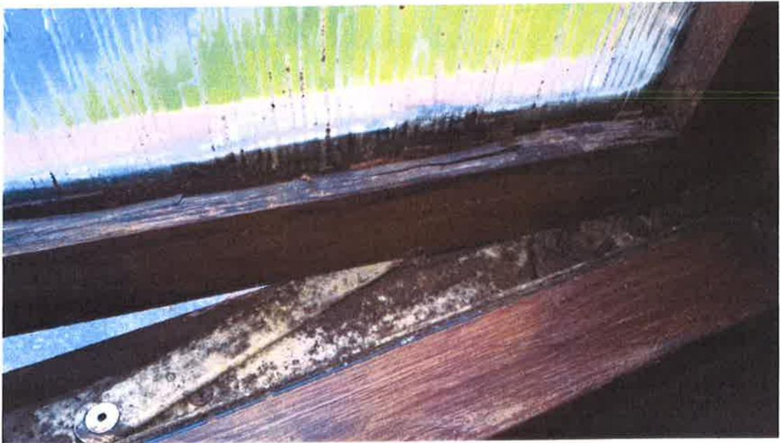
4. Close view of timber decay to window frame, defective glazing putties and water ingress at glazing seal.
