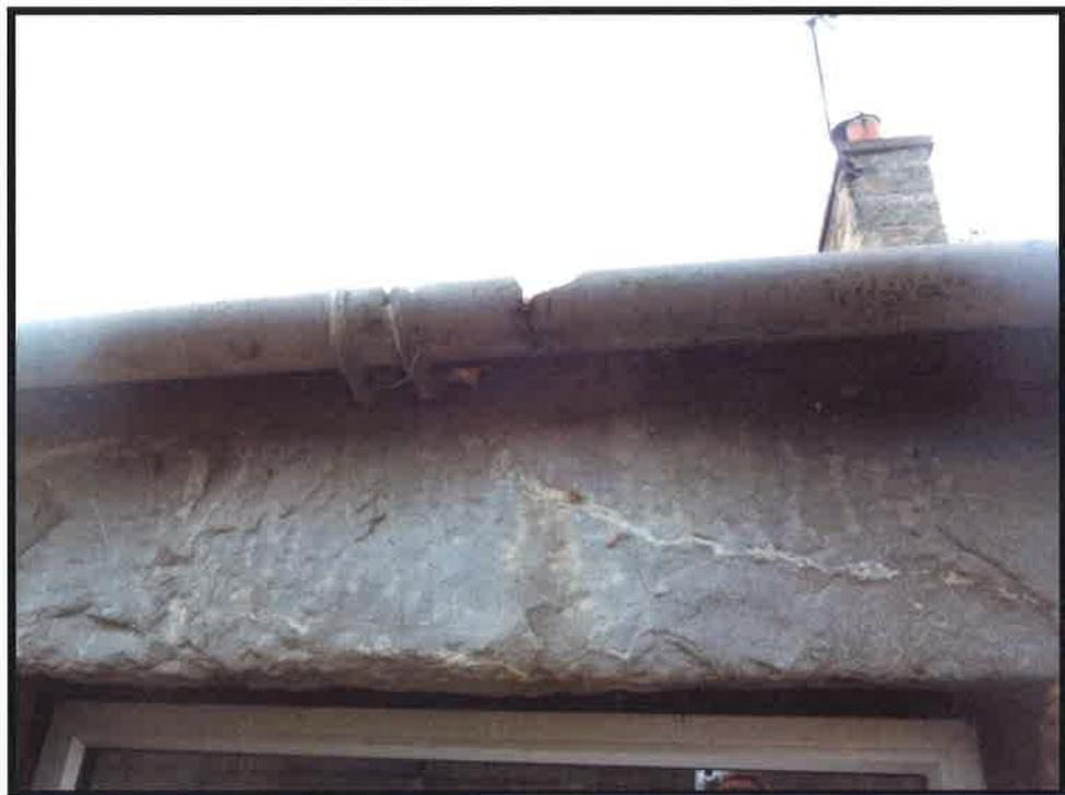
Figure 13 Broken gutter rear elevation
