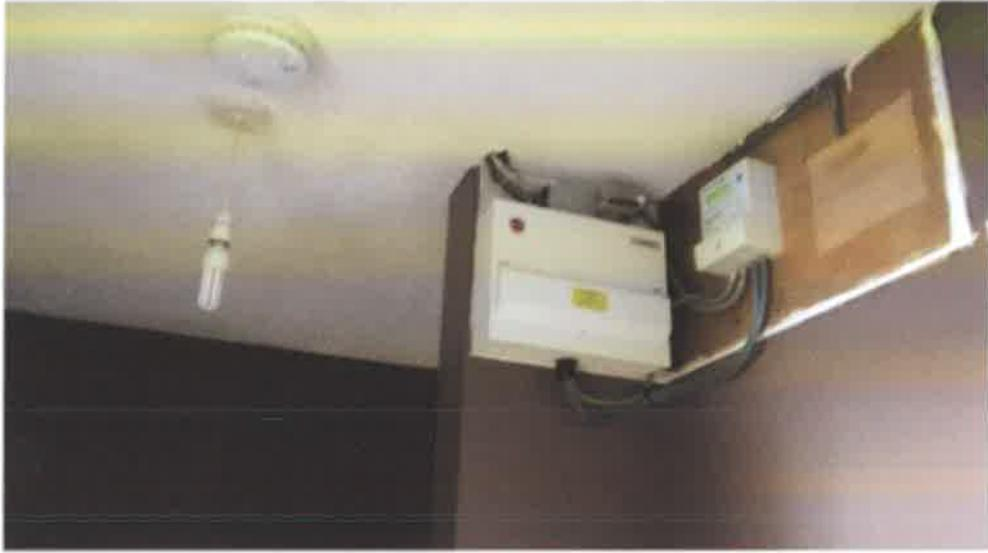
Photo 5: new electric consumer unit and upgraded fire detection system
