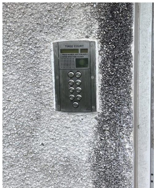
2. Security entrance buzzer (bottom left) on communal system serving flats 38-45
