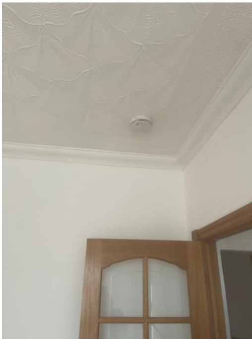
Photographs 10 and 11: smoke detectors to living room and hallway
