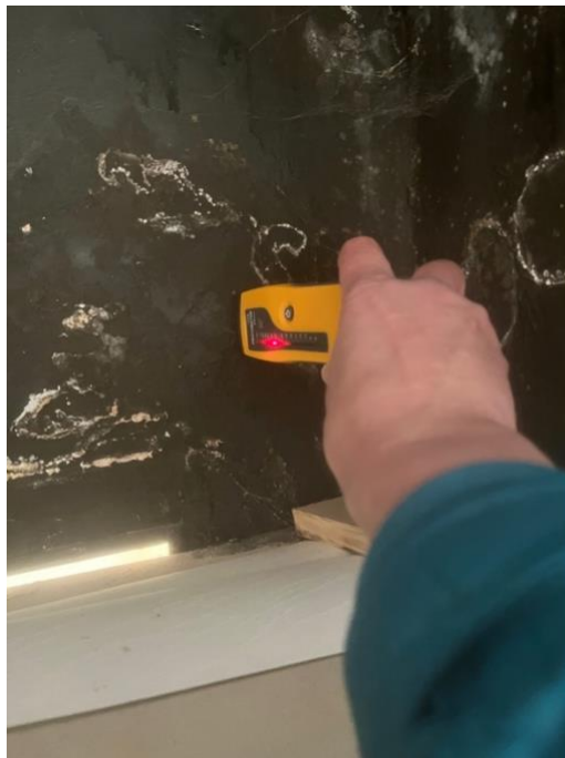
Photograph 7: Bedroom 1: to upper inside of wardrobe (indicating higher than normal levels of moisture)
