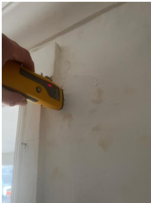
Photograph 5: Bedroom 1: to upper right hand side of window (indicating higher than normal levels of moisture)
