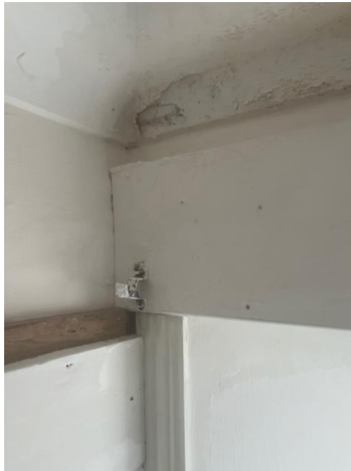
Photograph 7: Bedroom 1: to upper inside of wardrobe (indicating higher than normal levels of moisture)
