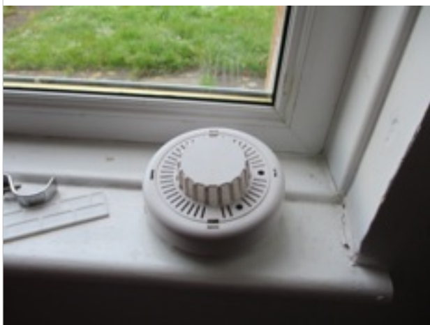
Heat detector loose/lying on living room window sill (observation)
