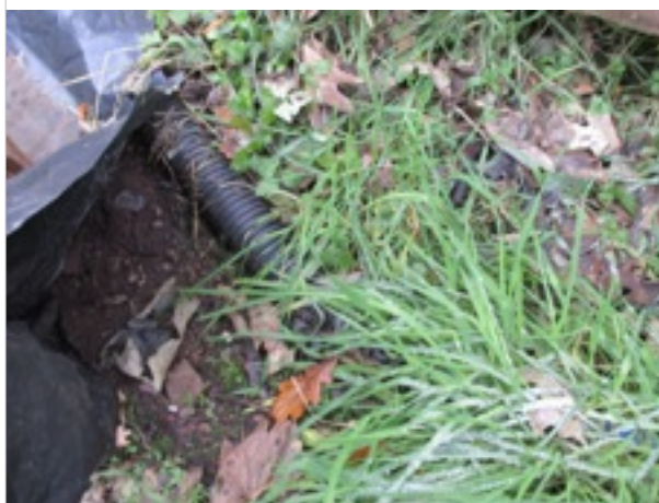
Back garden - exposed section of land drainage pipe at base of grassed slope just within southern boundary of garden
