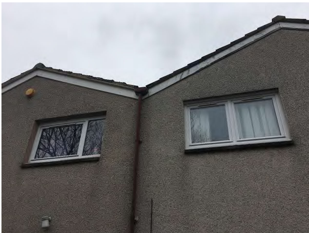
Rear elevation showing location of valley gutter
