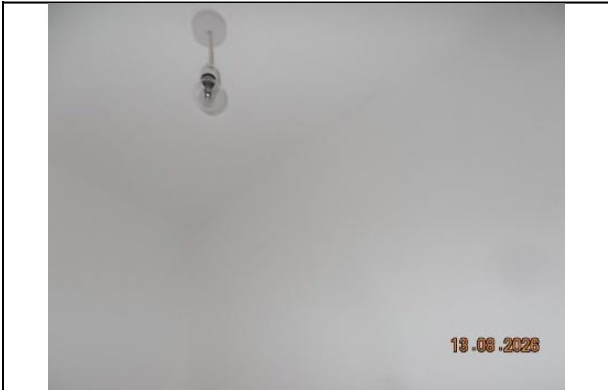
5. Ceiling of other cupboard off hallway
