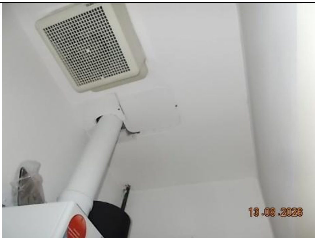
4. Ceiling of utility cupboard off hallway
