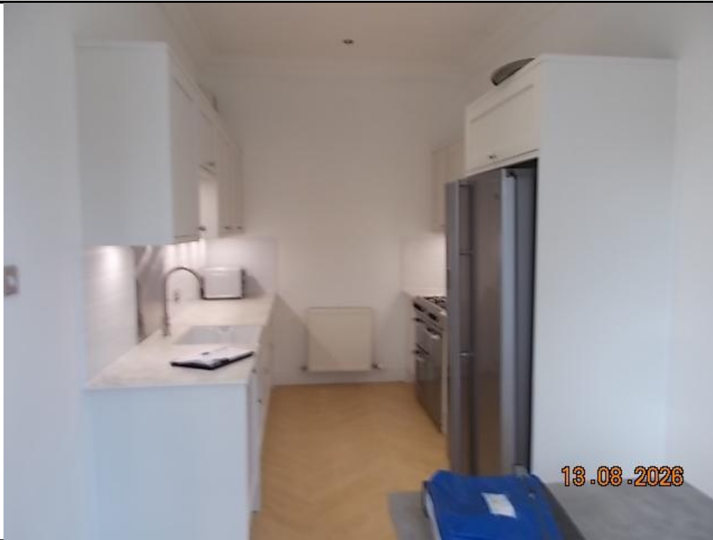
1. General view of kitchen recess
