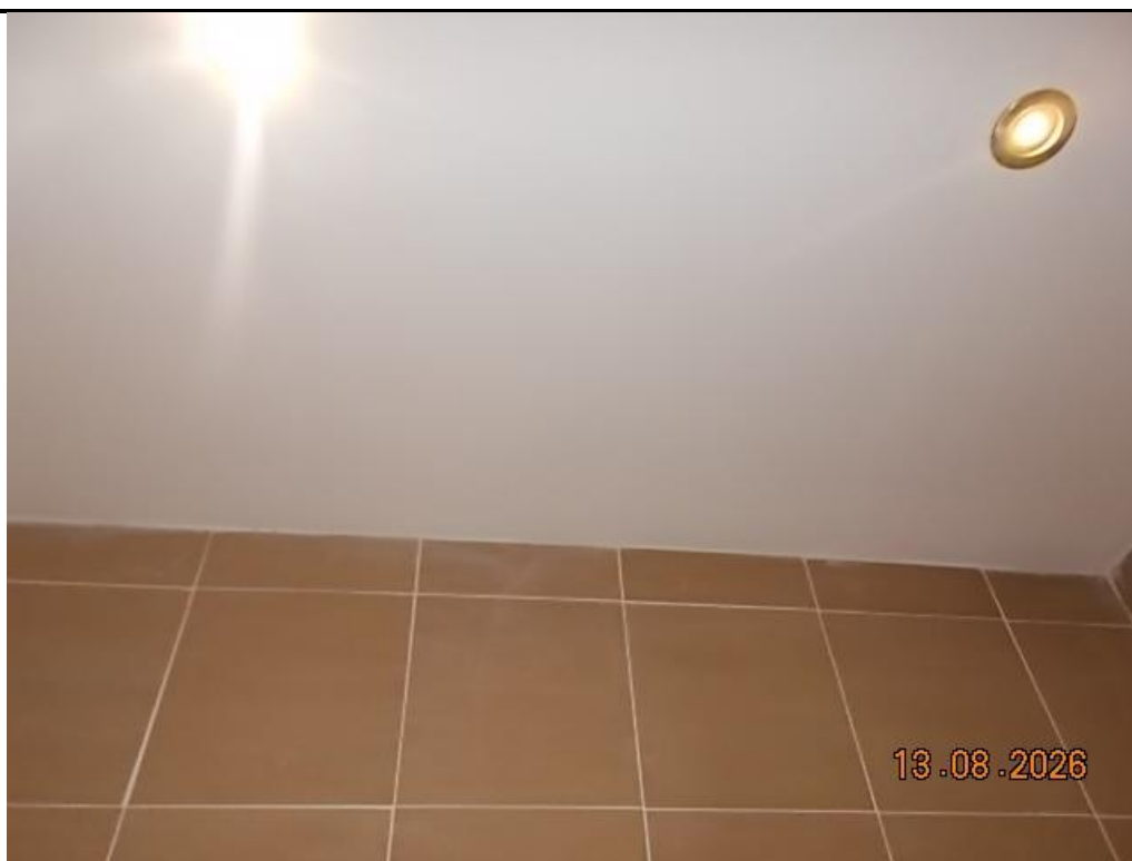
7. Ceiling of family bathroom
