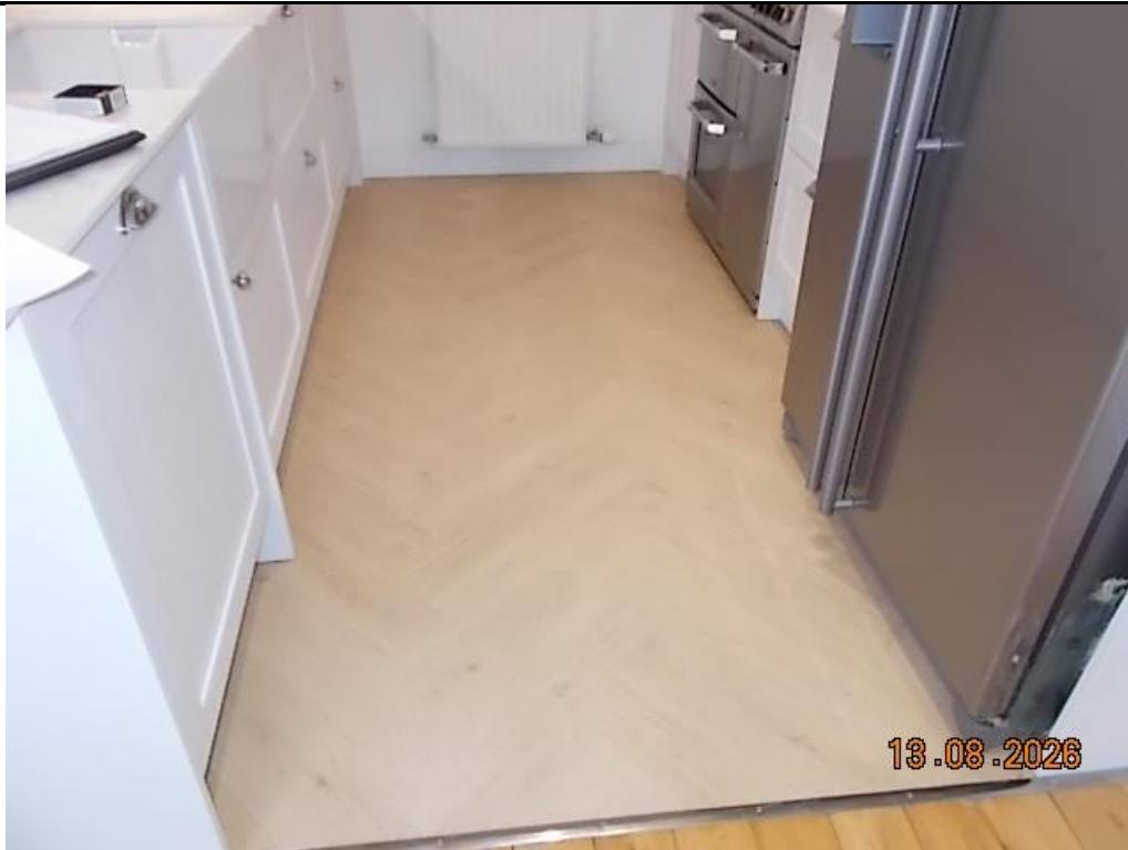
2. General view of floor to kitchen recess
