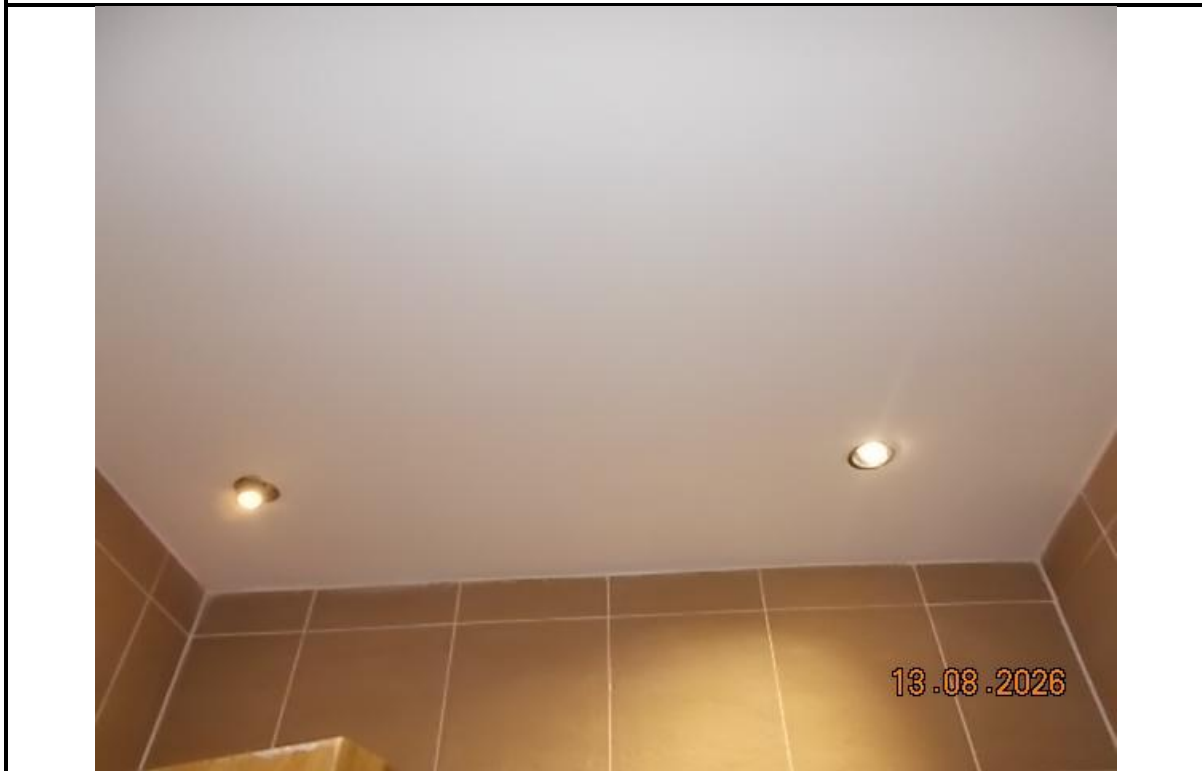
6. Ceiling of family bathroom
