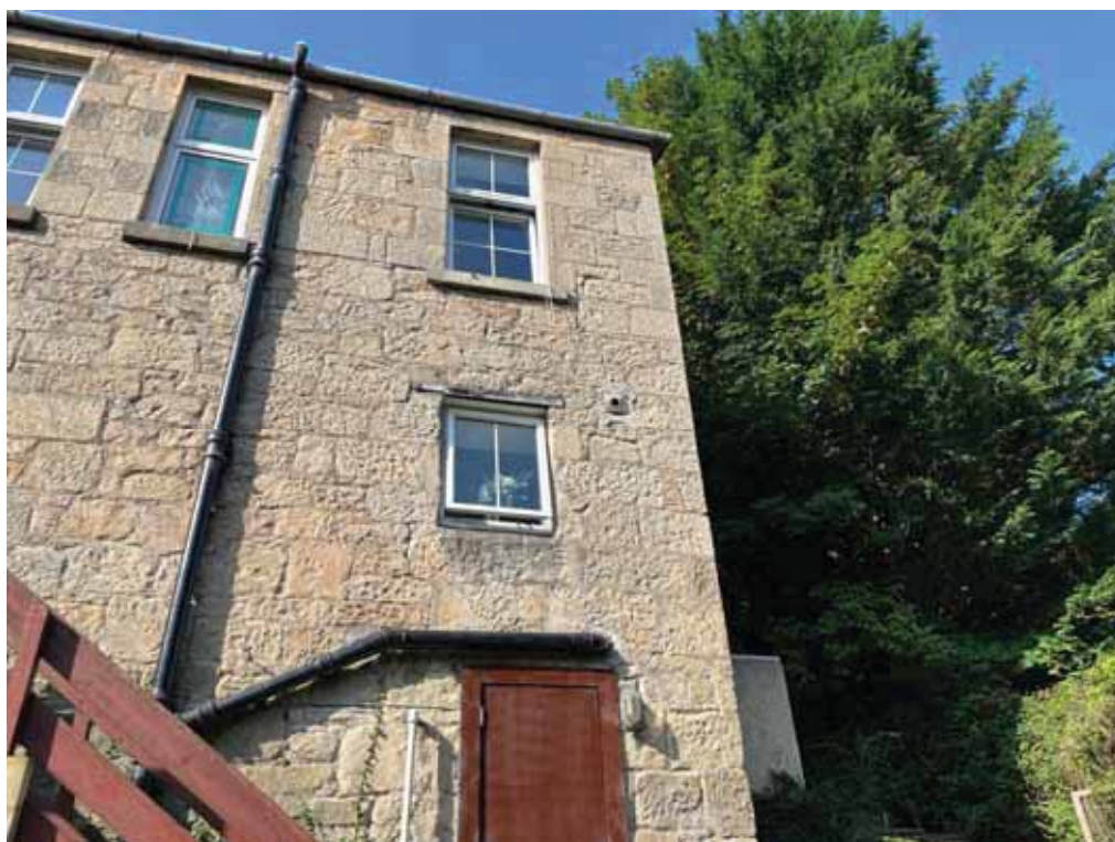
Exposed timber lintol
