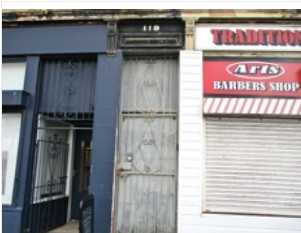
Common entrance door to pend accessing backcourt and subject property
