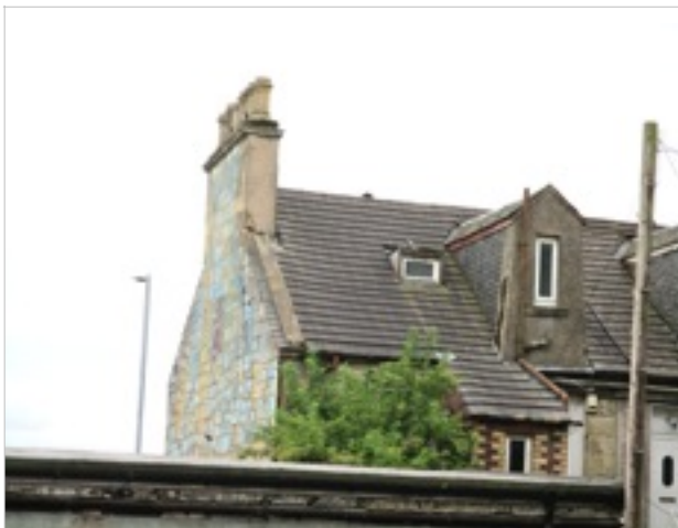
Rear elevation - view of roof to adjoining flat (119b) and gable wall
