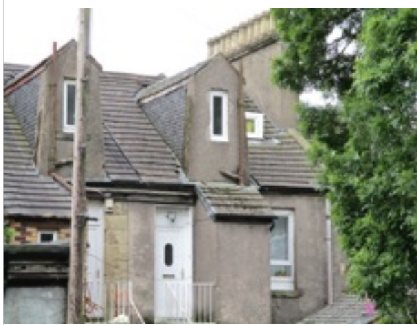
View of rear elevation and roof
