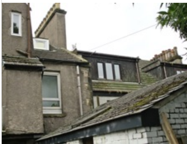
Rear elevation and pitched tiled roof/dormer windows and outbuilding
