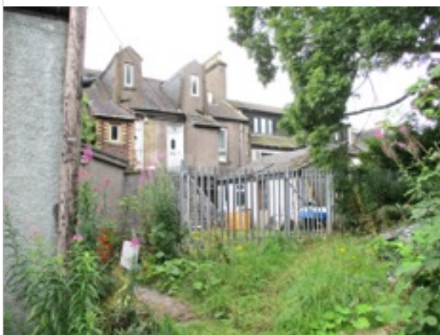
Rear view showing metal security fencing/no access gate
