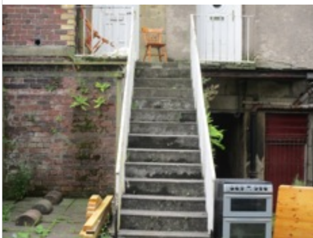
Rear elevation - common access steps leading to landing on back projection with front door of 119a on right side
