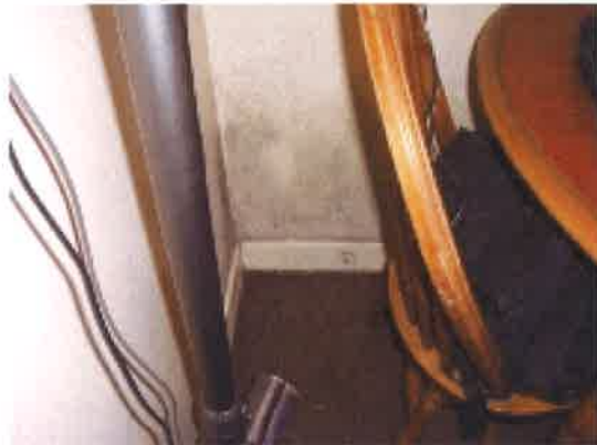
CONDENSATION MOULD IN DINING AREA
