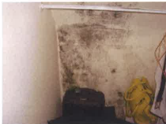
CONDENSATION MOULD IN BED CPD
