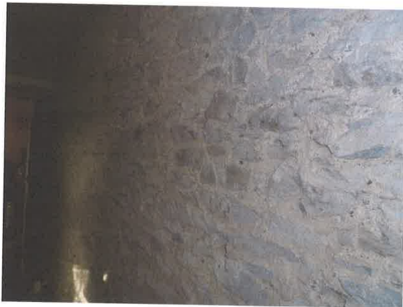
12. Wall stripped back at sitting room
