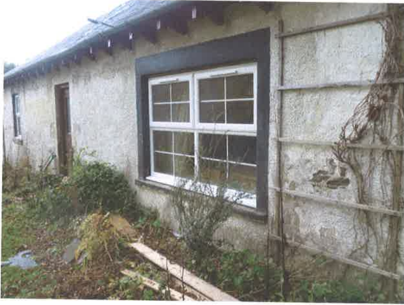
7. Replacement UPVC window
