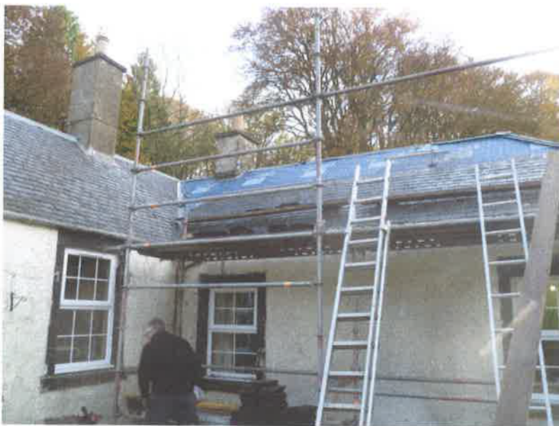
2. On-going work – north west elevation
