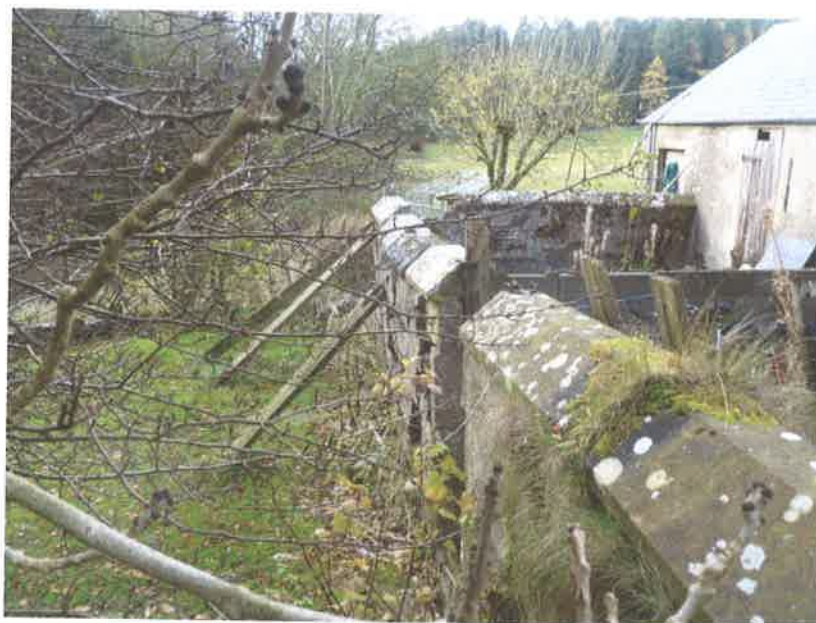
9. Wall at byre
