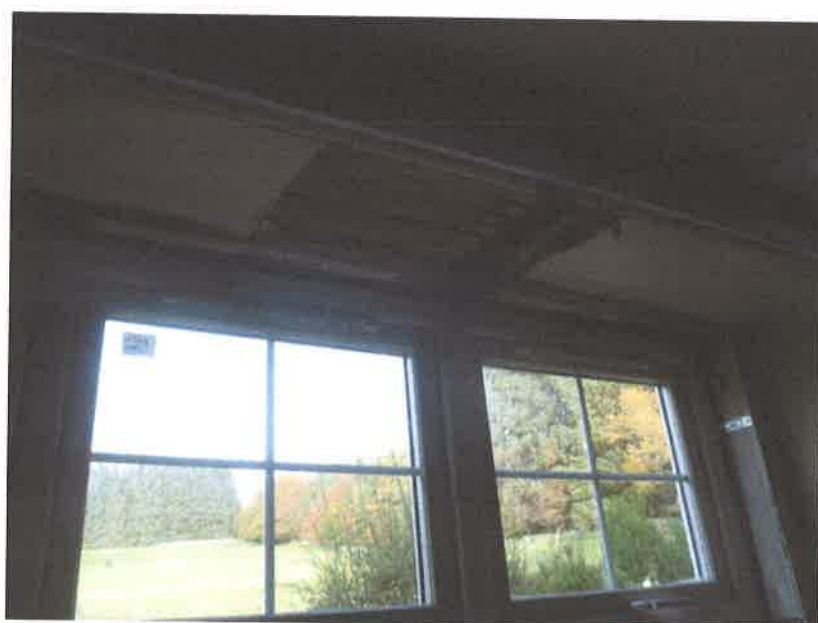
10. Replacement window internally at sitting room
