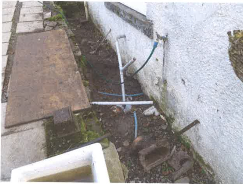
5. Water supply – lead replaced with alkathene
