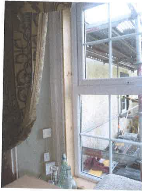
11. Window finishing internally
