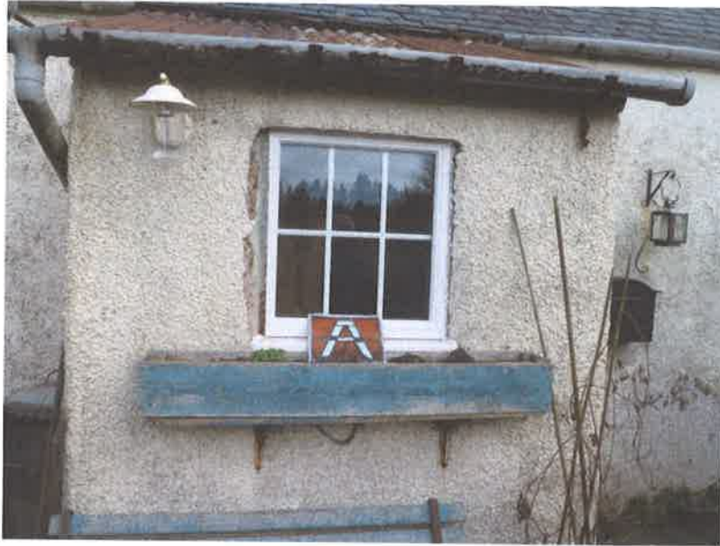
3. UPVC Replacement window - vestibule
