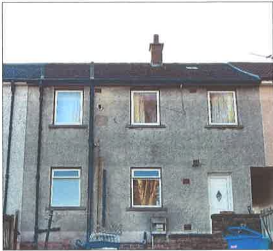
Holes in roof - No evidence of missing or broken tiles – heavy covering of moss at the rear elevation. No evidence of bird's nest at rear bedroom window
