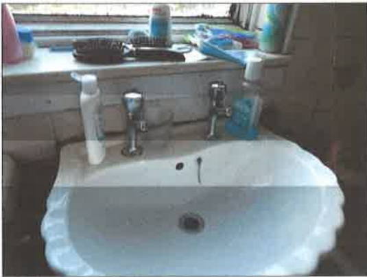
Loose leaking taps - New taps fitted
