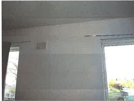
Dampness on walls and ceiling back bedroom – no evidence of water ingress Landlord cleared guttering and painted wall and ceiling.
