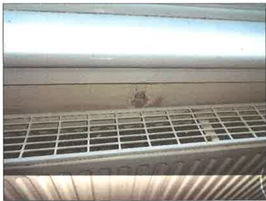
Crack below living room window
