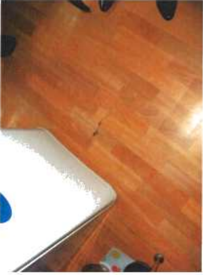
10 - Kitchen - damage to vinyl at loose flooring
