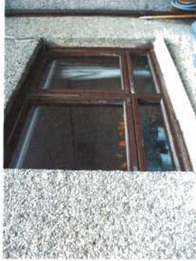
09 - Living room - window external
