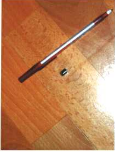
11 Kitchen - 'nailhead?' protruding from vinyl
