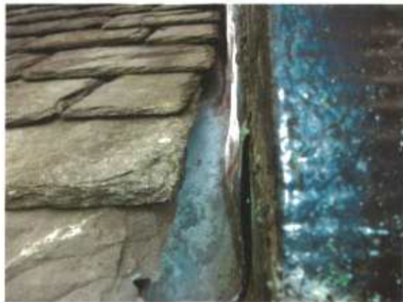
14 - External view of 13 (from front)
