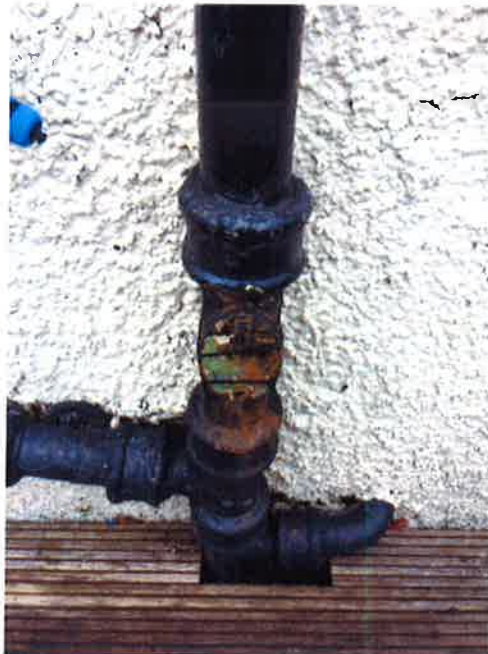
Soil stack – re-sealed
