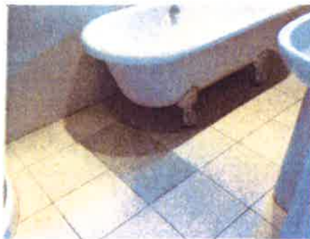
En suite replacement floor tiles 19 th June 2017
