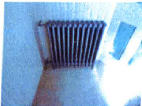
Bathroom Radiator 3 rd April 2017
