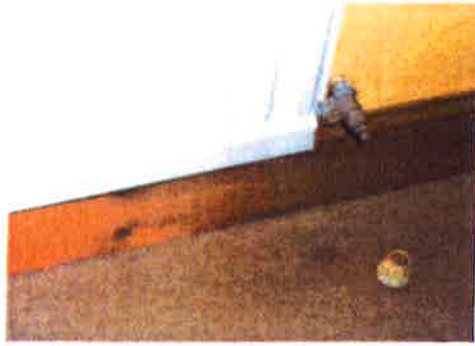
Dining Room Radiator 3 rd April 2017
