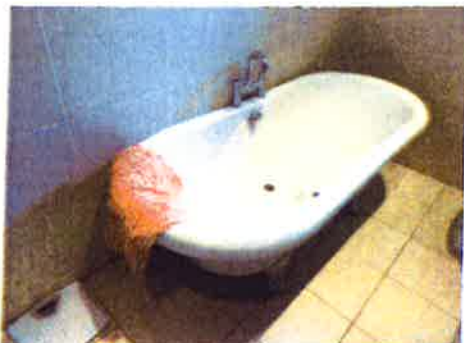
En suite original floor tiles 3 rd April 2017
