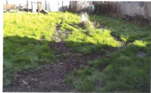
Photo 5 – Septic tank soakaway
