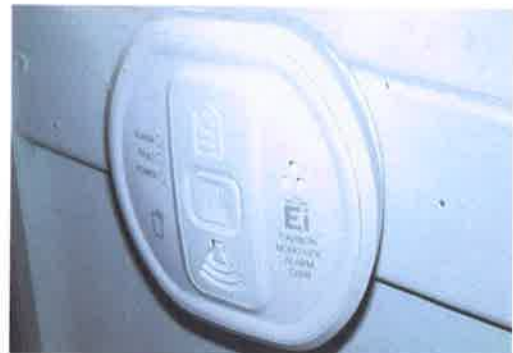
Photo 7 – Carbon Monoxide alarm
