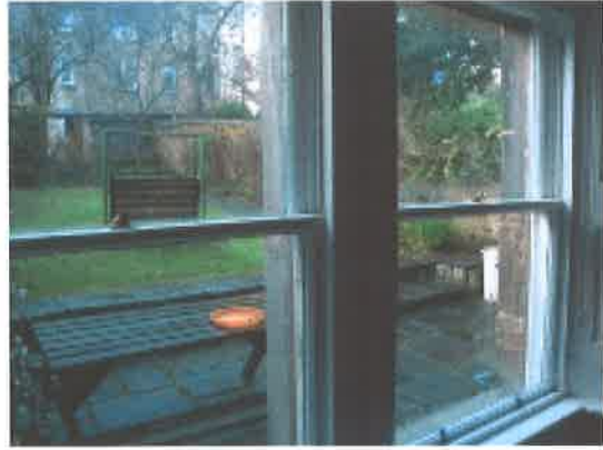
Windows in LR properly closed.
