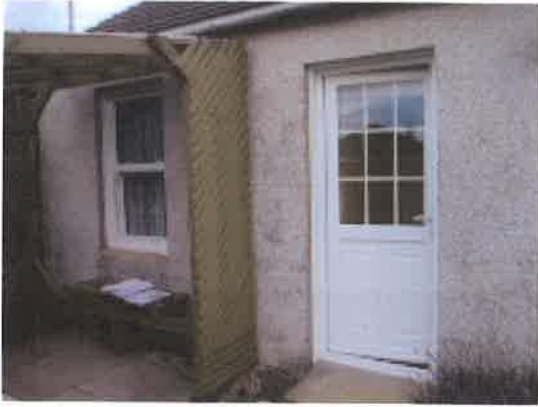
Rear elevation – new window.
