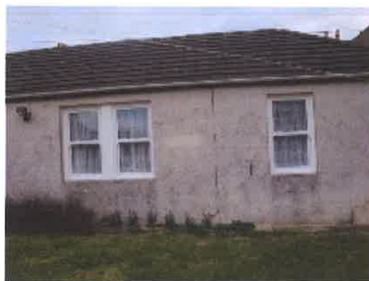
Rear elevation – new windows.
