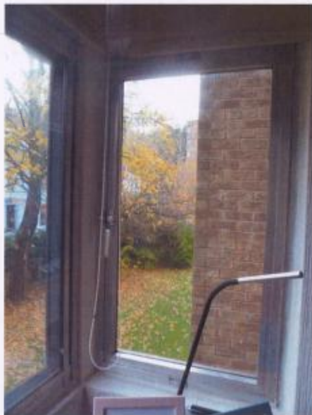
8. Window – living room
