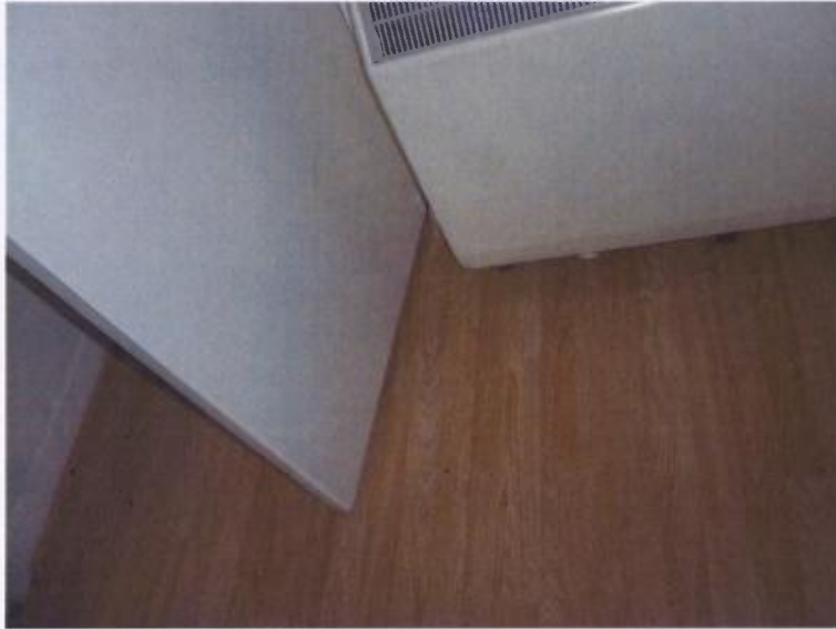
3. Storage heater – living room
