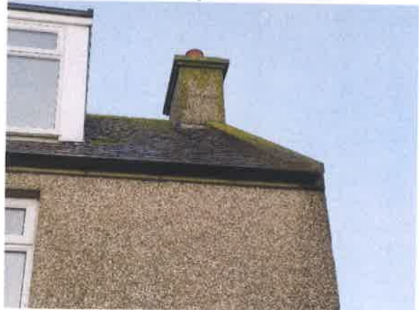
12 Skew abutment detail.
