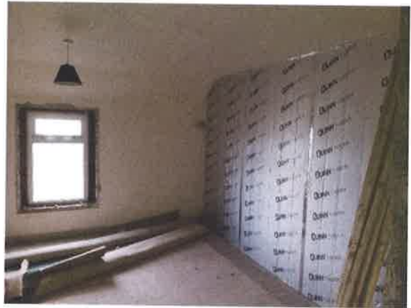
8 Refurbishment works ongoing including additional insulation.
