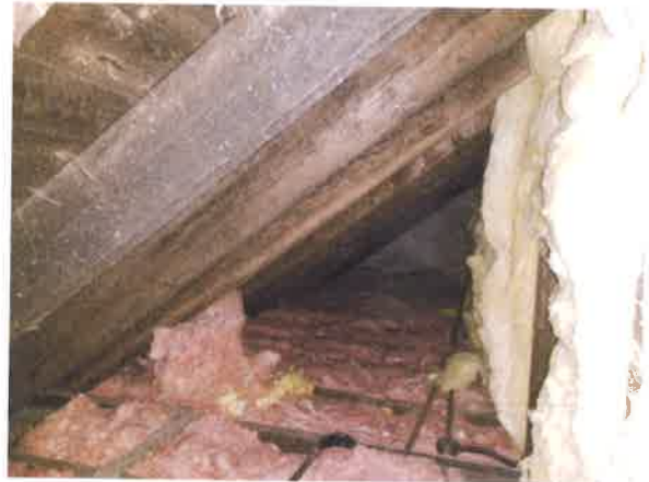
10 Eaves void and existing insulation levels.
