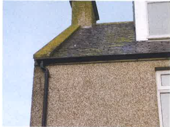
14 Skew abutment detail.
