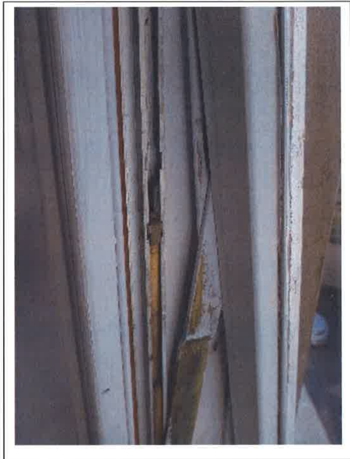
Internal windows showing draught proofing
