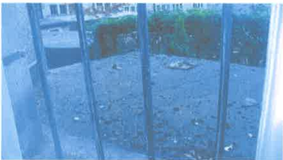
Photo 12 Flat roof above kitchen extension
