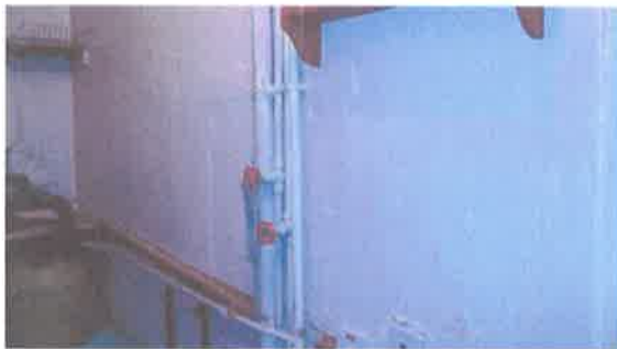
Photo 4 Saturated wall – L/R cupboard
