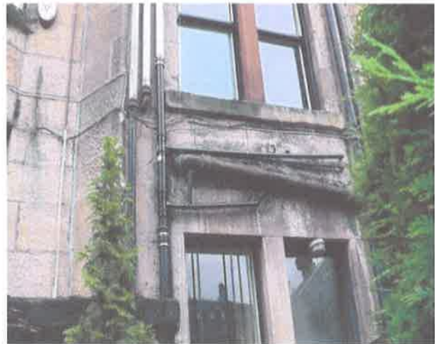
Photo 17 Recently replaced pipework at rear
