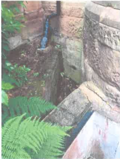
Photo 16 Rainwater run-off front elevation
