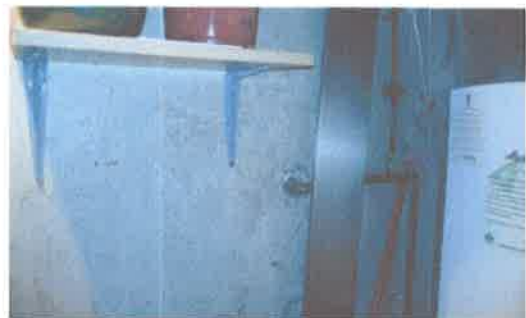
Photo 5 Damp wall – boiler cupboard
