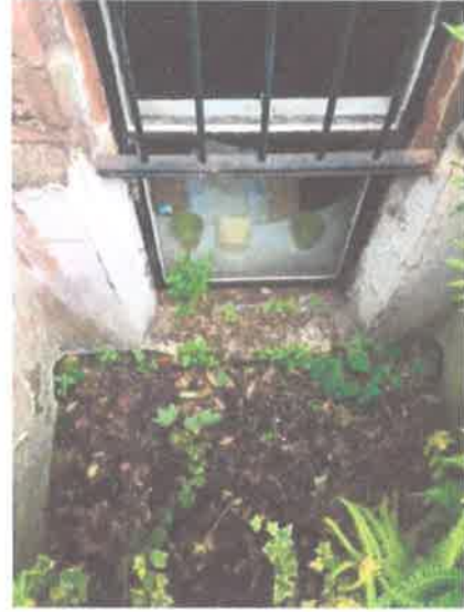
Photo 15 Ground build-up at front bed.
