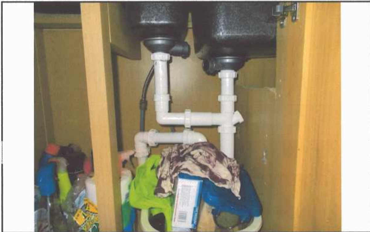
3. Drainage Below Kitchen Sink
