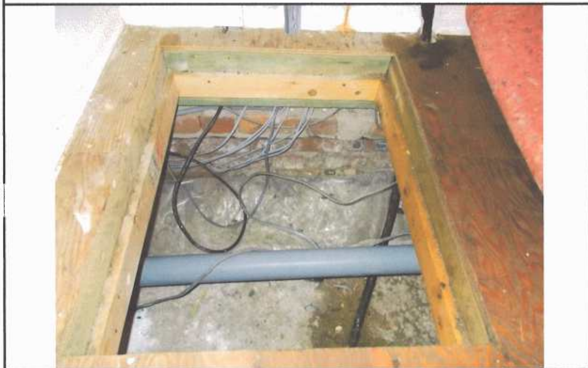
4. Solum viewed from hatch in floor in Understair Cupboard
