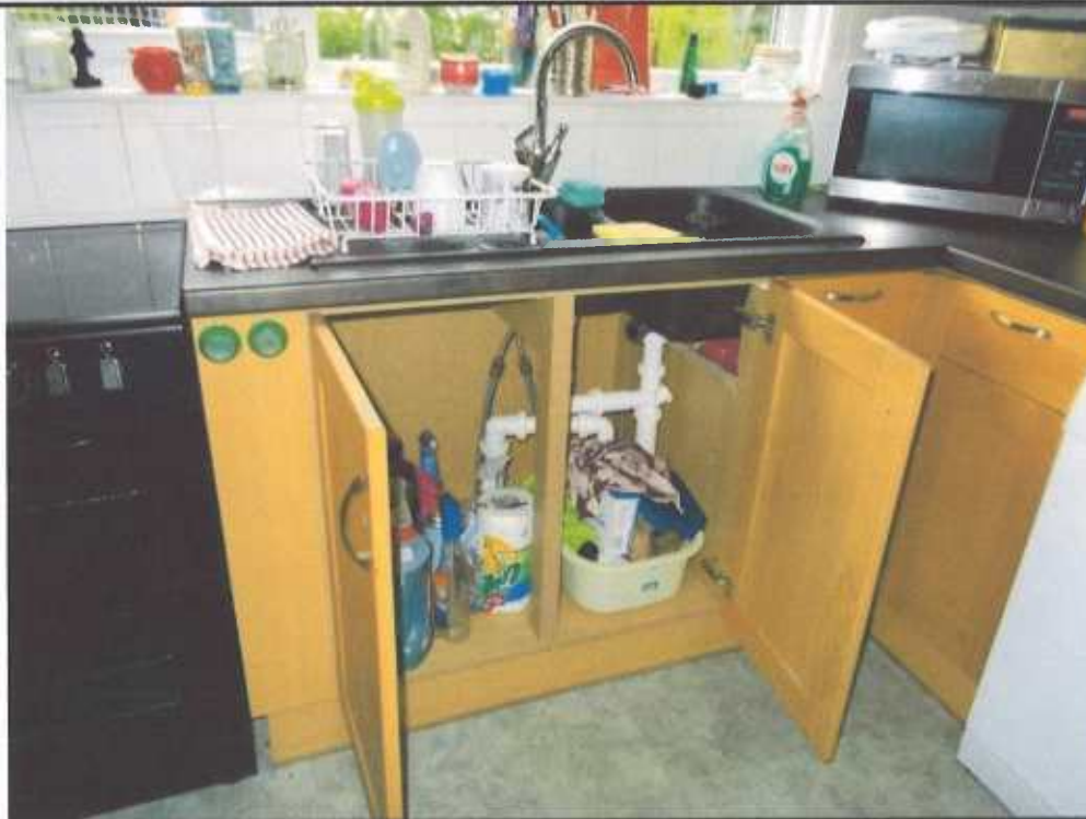
2. Drainage below Kitchen Sink
