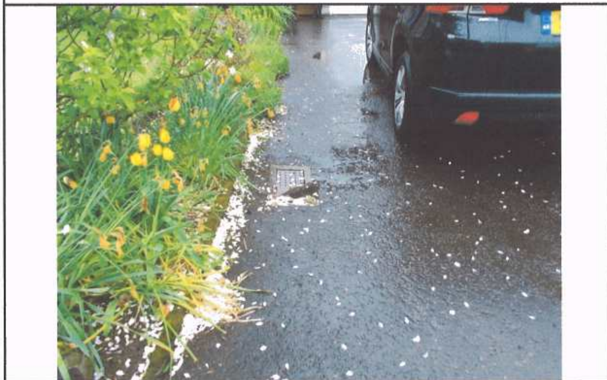
8. Cover on line of drain in driveway at front of property
